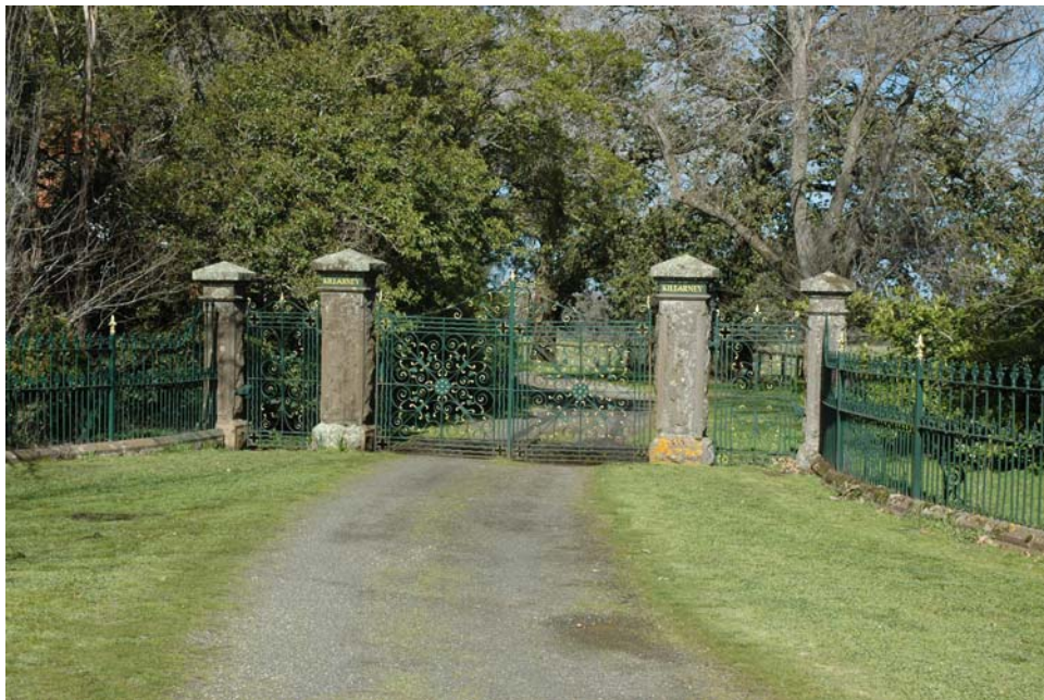
Illustration 3 Gates at Killarney, Dunnstown, 1901 have a similar scale and layout but differ in detail and cast iron pattern. They were designed by George Clegg, architect of Ballarat, who had also designed James Coghlan's home in Ballarat in 1888 and if the gates date from Oswald Coghlan's ownership may possibly have been the architect. 17
