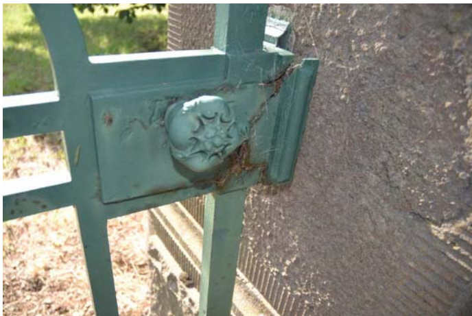
Photo 3 Detail of lock and cast iron handle
