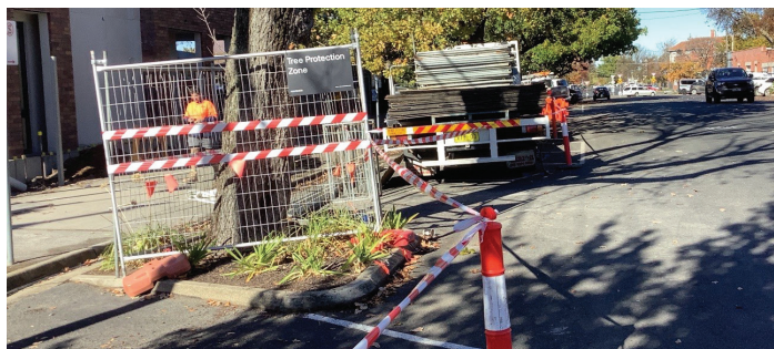
Figure 5 - Tree Protection Zone does not meet AS 4970-2009 and City of Ballarat Guidelines
