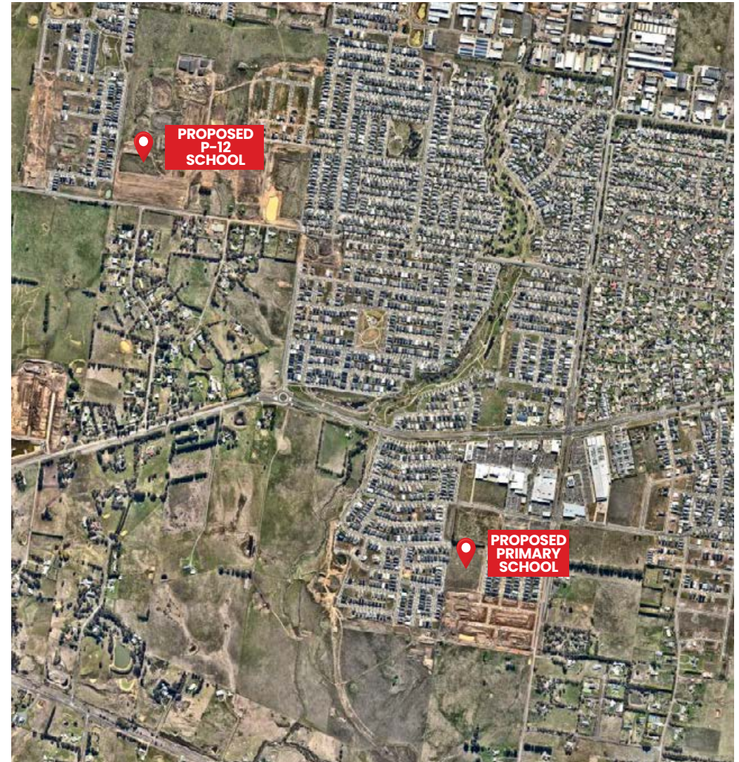
Site Aerial as of August 2025
