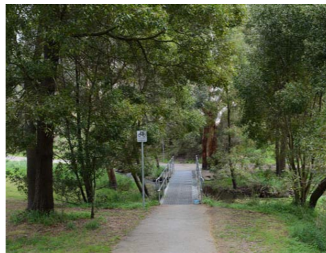
Typical northern reach bridge
