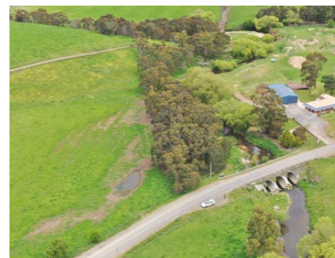
Nolans Road Bridge
