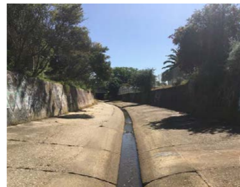
Northern end of channelised section of Yarrowee River. Concrete channel.
