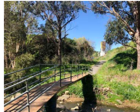
Tannery Lane pedestrian bridge
