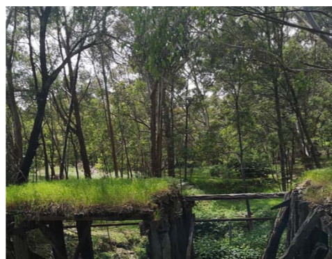
Henderson Lane Bridge and bushland
