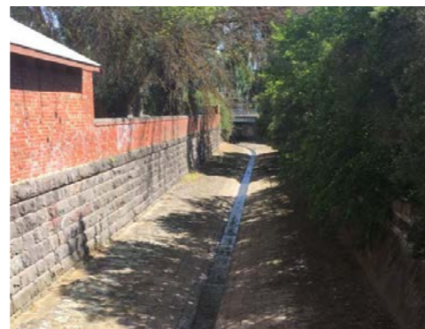
Bluestone channel through Eastern Oval. Oval facilities are fragmented by the channel.
