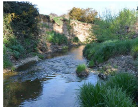
Erosion of CHW treatment plant pond bank
