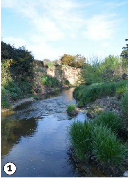
1 Erosion along CHW treatment pond bank
