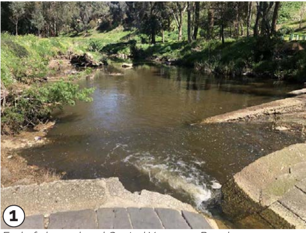
1 End of channel and Central Yarrowee Reach
