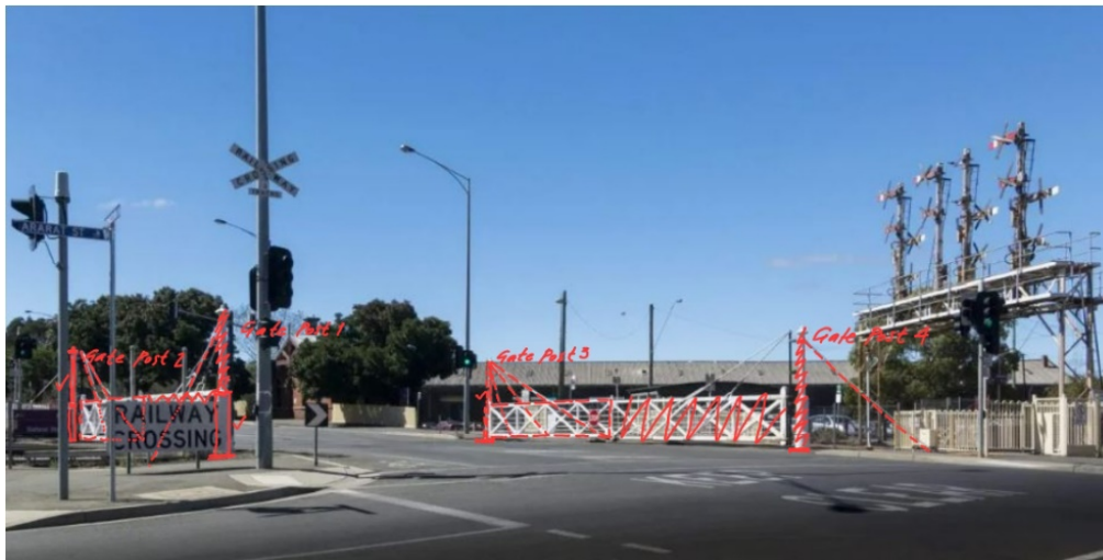
Figure 1. Part of a street view prior to 20 May 2020 looking northeast to the Lydiard Street North Interlocking Sector Gates showing location of gate parts.
