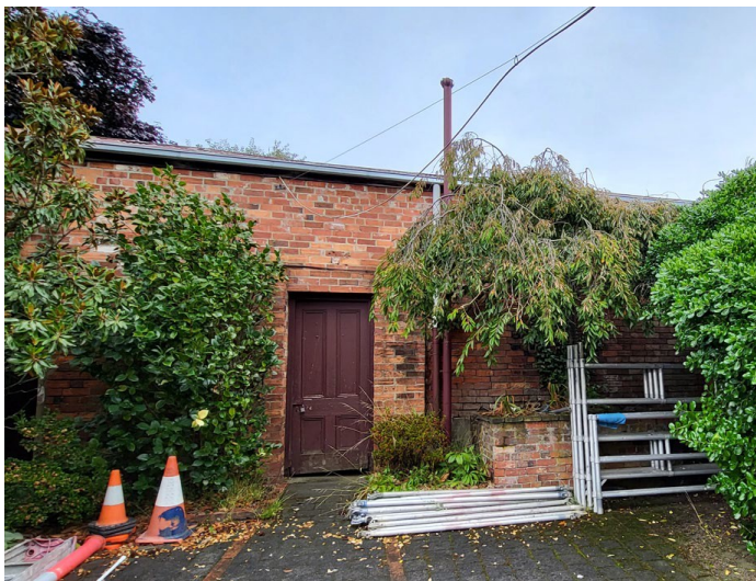
Figure 20. Four-panel pedestrian door to the north part of the stables. (Landmark Heritage, 2023)
