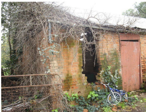
Figure 29. Plough Inn stables in 2009. (Heritage Victoria, 2009)
