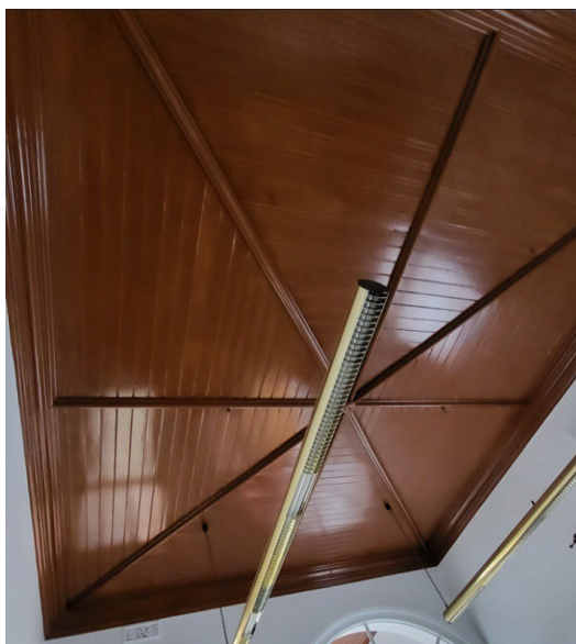
Figure 17. Timber-lined ceiling in the former Main Bar. (Landmark Heritage, 2023)
