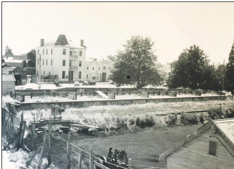
Figure 7. A view of the Carriers' Arms Hotel from the market reserve (now Civic Hall site), c1930s. The men's toilet block is visible at the rear. (Source: Ballarat Library cited in Ballarat Revealed)
