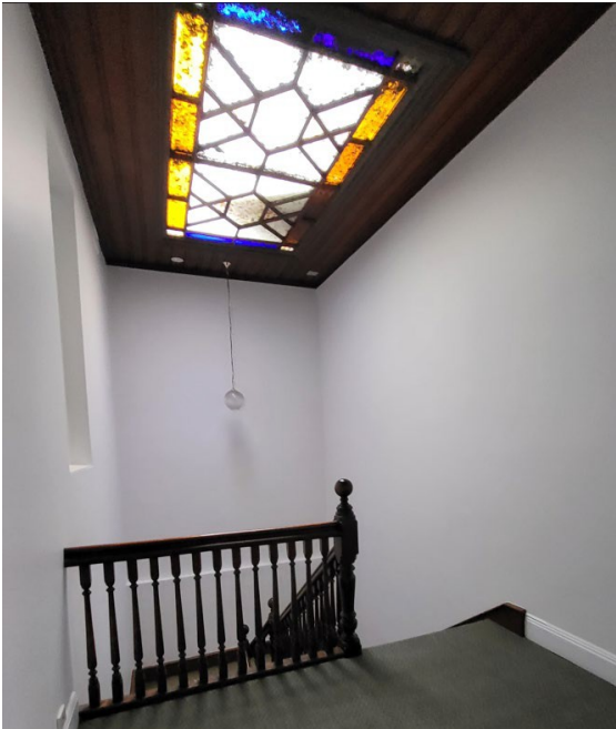
Figure 18. Top flight of the staircase and associated skylight. (Landmark Heritage, 2023)
