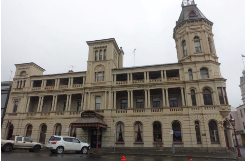
Figure 24. Front of Craig's Royal Hotel. The left-hand loggias and flanking towers date to 1862, while the right-hand loggias and hexagonal corner tower are from 1890. (Landmark Heritage, 2023)
