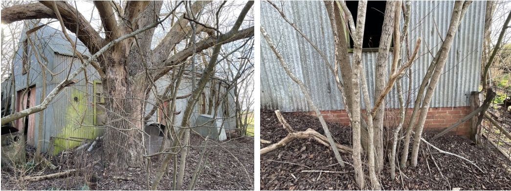
(Left) Rear (east) elevation showing the double carriage doors and window above in the south end wall (Right) Section of east wall at the north end showing the brick footing.
