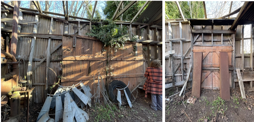
(Left) Double ledged carriage doors in the south wall. Note metal farm windmill parts and remnant plant at left (Right) Double ledged and braced doors in the south wall
