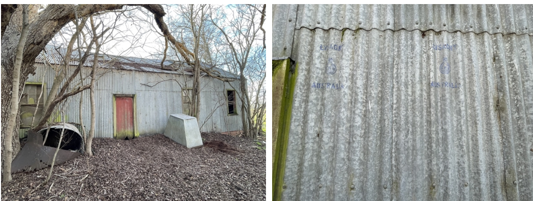
(Left) Rear (east) elevation (Right) 'Lysaght Australia' stamps on the iron to the right of the door in the image to the left.
