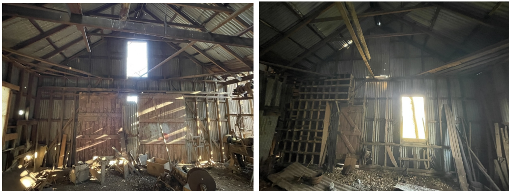
(Left) South end of rear section showing double ledged carriage doors, window above and remnant equipment at right (Right) North end of rear section showing ledged and braced door, window and pigeonhole shelving
