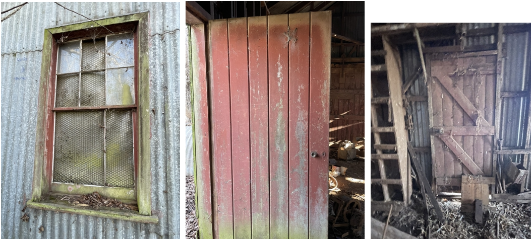
(Left) Typical window (Middle and right) Typical ledged and braced timber doors.
