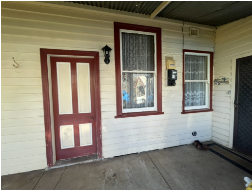
(Left) The door in the south wall added to provide access to the post office room. The window beside is original, while the window on the far right was added c.1950s when the kitchen addition was built. (Right) Wrought iron front gate
