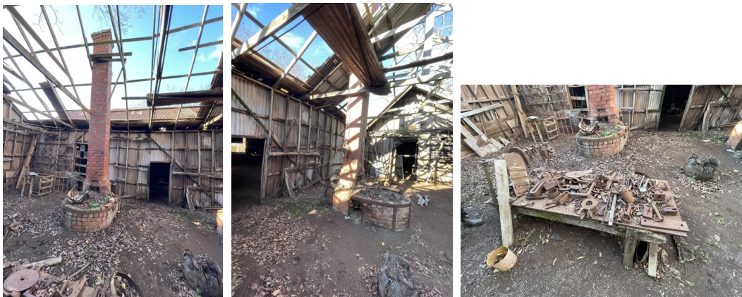
(Left and middle) The two forges in the south section also showing missing roof (Right) Low table strewn with tools
