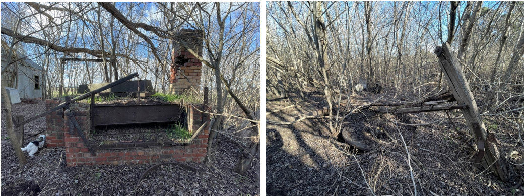
(Left) Wheel furnace at rear of building (Right) Wheel well and remnants of winch/crane beside the furnace
