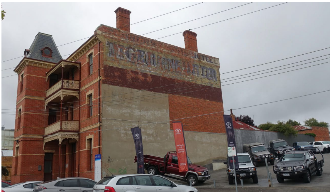
Figure 15. Hotel viewed from the north-east, with the painted signage visible at parapet level. Rising damp is visible at the base of this wall. (Landmark Heritage, 2023)
