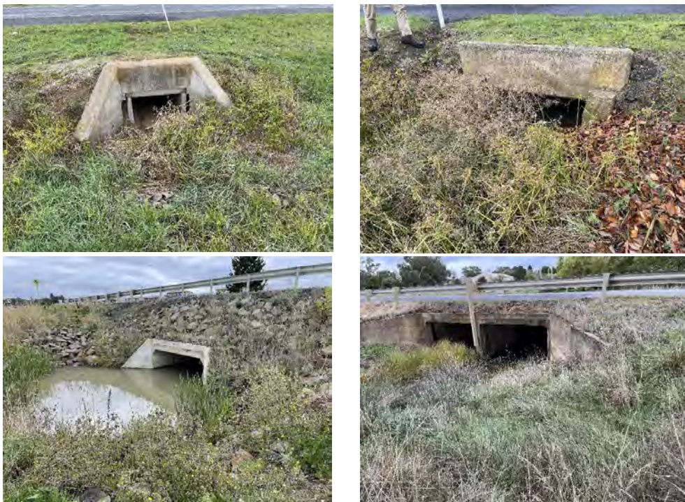
Figure 12. Photo of a typical road crossing of the waterway in the North-west growth area
