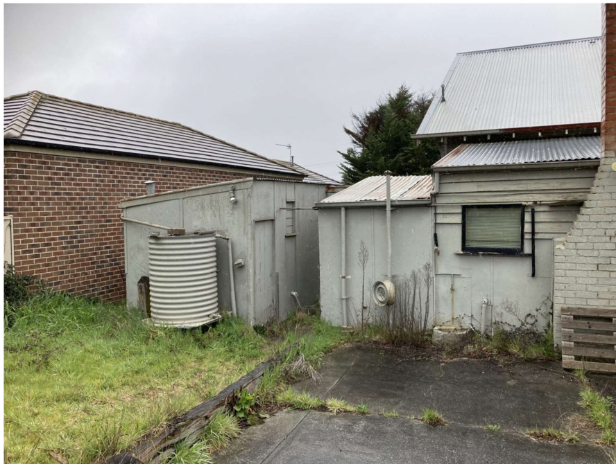
Figure 6 View to outbuilding north east of dwelling from rear yard, also showing c.1933 skillion kitchen and brick chimney.
