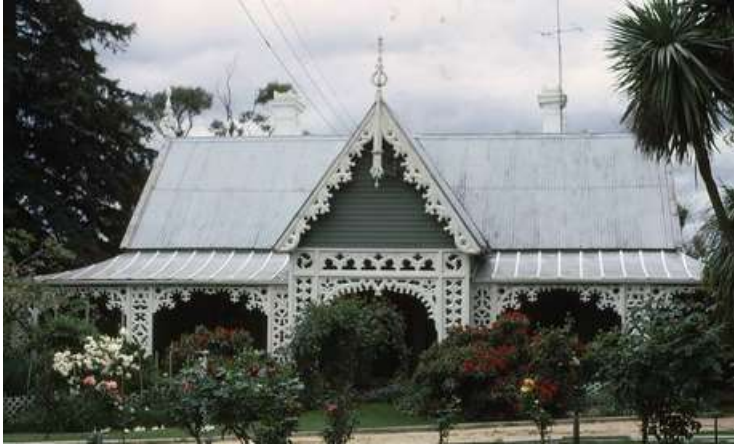
Figure 22. Ballantrae, Buninyong. Note the elaborate Gothic bargeboards and openwork verandah posts. (National Trust, n.d.)
