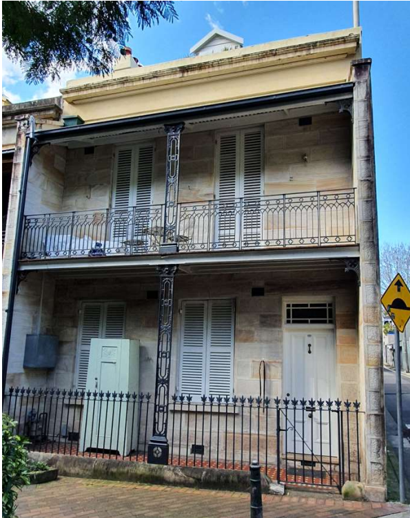
Figure 21. Terrace house in Darlinghurst, Sydney, with cast-iron pilasters produced by PN Russell. (Landmark Heritage, 2022)
