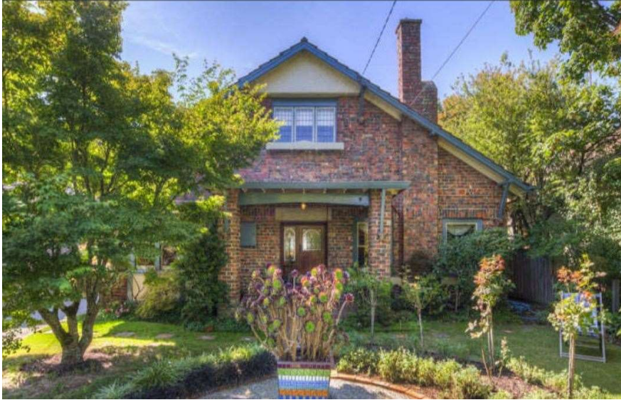
HO164 1505 Sturt Street, Newington. A large Arts & Crafts house of 1925 with single- and two-storey volumes. The base of the house is of clinker brick, with unpainted roughcast render above. The front fence is executed in matching materials. The single-storey section has an arched porch entry. The two-storey gabled section beside it has a timber-shingled apex. Casement and double-hung windows feature a triangular motif:
