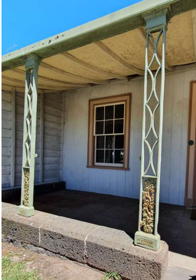
Figure 19. Cast-iron openwork verandah posts at Mills Cottage, manufactured by R Dawson, Sydney. (Landmark Heritage, 2021)
