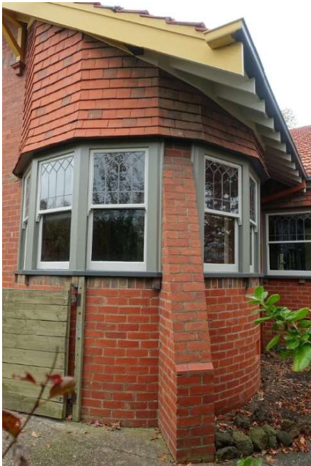
Figure 8. Circular, buttressed bay window at the south-west corner. Note hung terracotta tiles above it. (Landmark Heritage, 2022)
