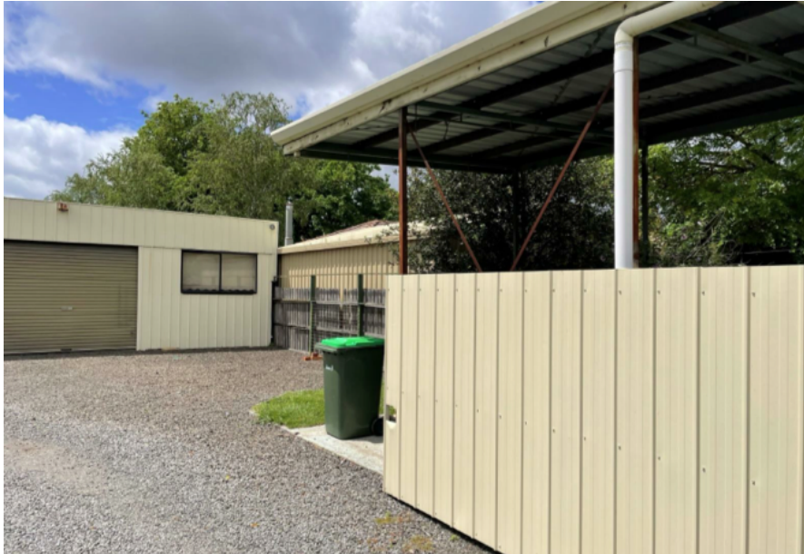
Figure 5 – rear of existing site
