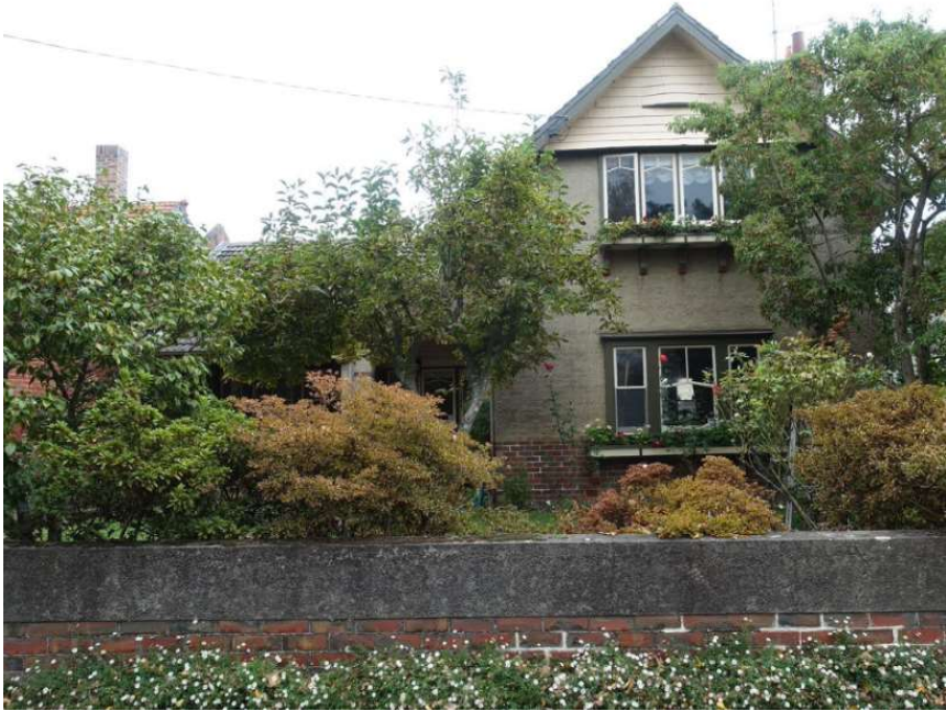
HO164 1505 Sturt Street, Newington. A large Arts & Crafts house of 1925 with single- and two-storey volumes. The base of the house is of clinker brick, with unpainted roughcast render above. The front fence is executed in matching materials. The single-storey section has an arched porch entry. The two-storey gabled section beside it has a timber-shingled apex. Casement and double-hung windows feature a triangular motif:
