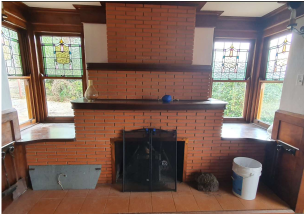
Figure 10. Detail of the orange-brick fireplace in the east front room. (Landmark Heritage, 2022)
