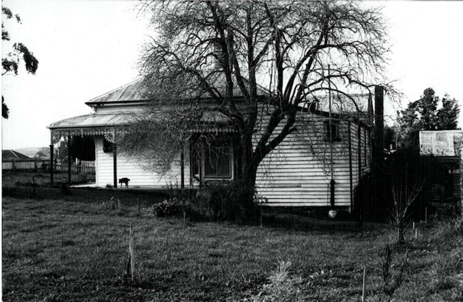
Figure 5. The south-west side elevation of subject property in 1972-73 before renovation. Note the return verandah, bay window and rear lean-to. (Photos by Peter Cuffley 1972-73)
