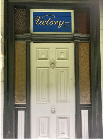
Figure 5 Early front door and surrounds with 'Victory' lettering
