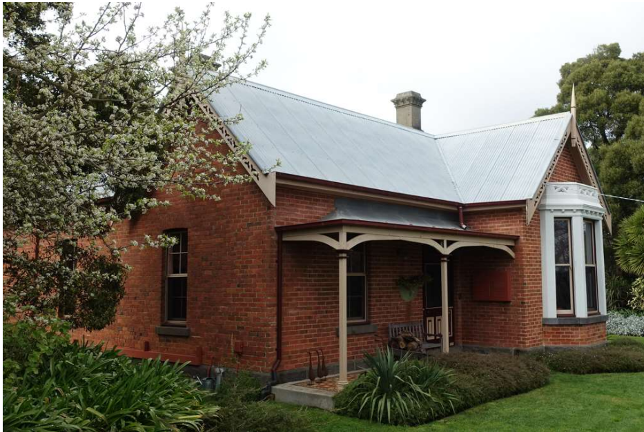
Figure 9. Front section of the former Parsonage, showing the two gables and one of the rendered chimneys. (Landmark Heritage, 2022)
