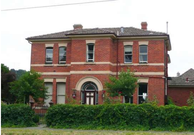
Figure 17. Former Female Refuge. (Heritage Victoria, 2008)
