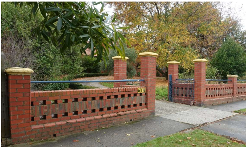
Figure 13. Front brick fence and vehicular gateway. (Landmark Heritage, 2022)
