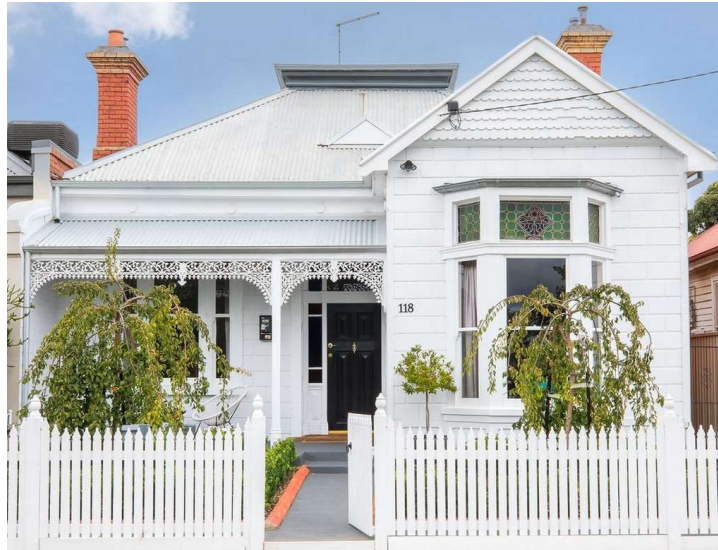
Figure 17. 118 Victoria Street, Ballarat East. Note the flat platform atop the roof. The verandah has been rebuilt. ( www.realestate.com.au , 2021)
