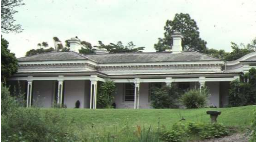
Figure 18. Glenara, Bulla, built c1857. (Heritage Victoria, 1983)
