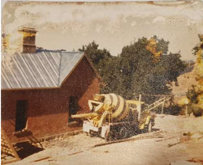
Figure 4. The former Parsonage undergoing works c1981. Note the new roofing, windows removed, and mixer pouring a concrete floor. (Collection of C & M Sargent)
