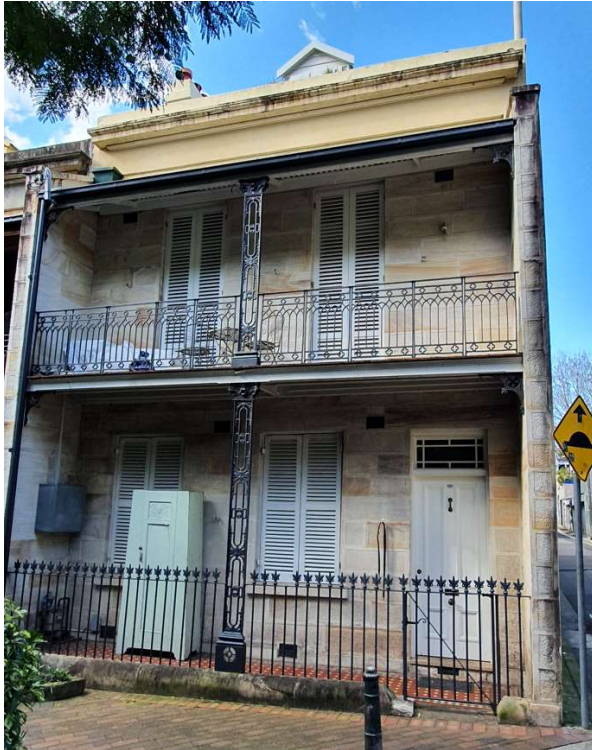
Figure 21. Terrace house in Darlinghurst, Sydney, with cast-iron pilasters produced by PN Russell. (Landmark Heritage, 2022)
