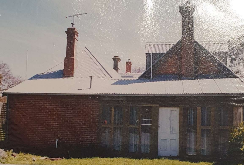
Figure 6. East (rear) elevation of former Parsonage in 2000, prior to demolition of the timber-framed part of the rear lean-to (at right). (Collection of M & C Sargent)
