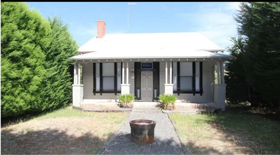
Figure 1 Facade 'Victory' house
