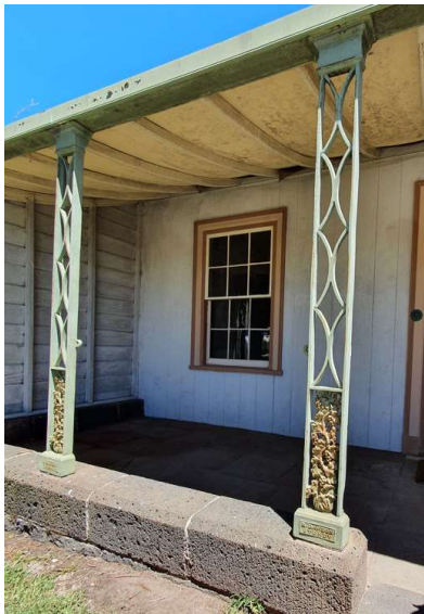
Figure 19. Cast-iron openwork verandah posts at Mills Cottage, manufactured by R Dawson, Sydney. (Landmark Heritage, 2021)
