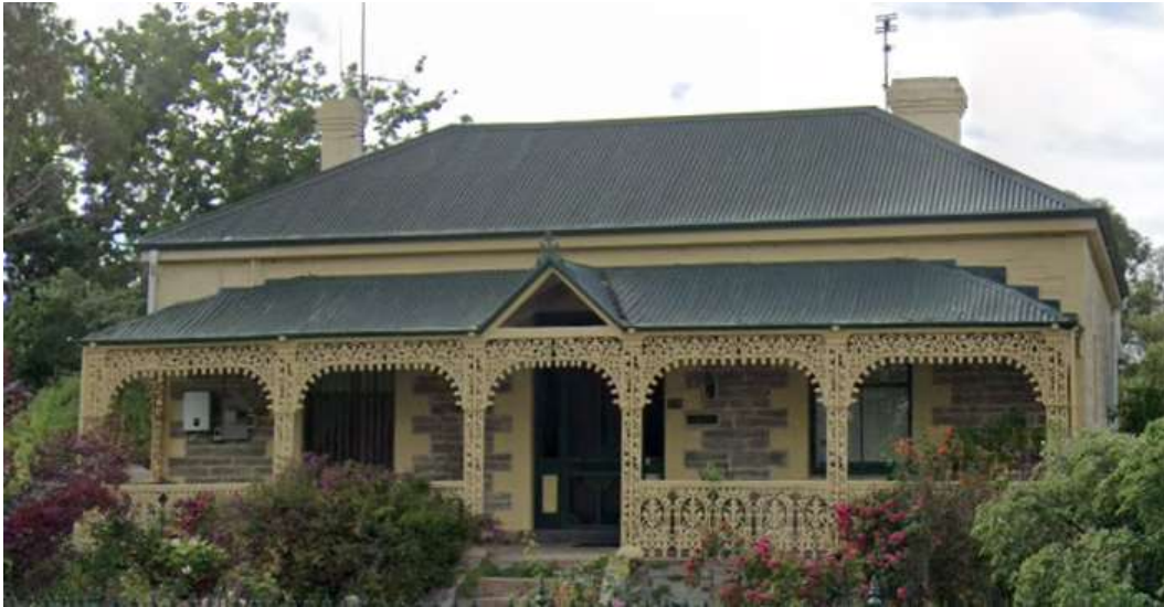
Figure 23. Nyora, 59 Victoria Street, Eaglehawk (Bendigo). (Google Streetview,
