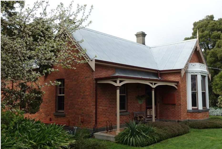
Figure 9. Front section of the former Parsonage, showing the two gables and one of the rendered chimneys. (Landmark Heritage, 2022)
