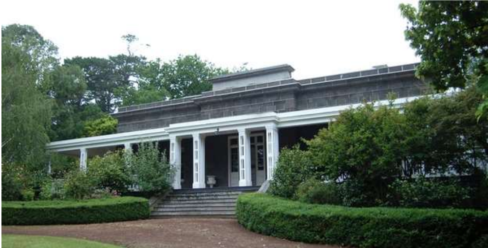
Figure 17. Maretimo, Portland North, built c1854. (Heritage Victoria, 2008)
