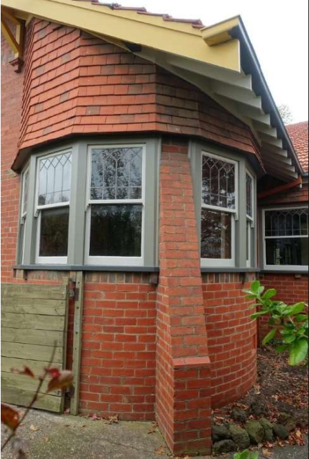
Figure 8. Circular, buttressed bay window at the south-west corner. Note hung terracotta tiles above it. (Landmark Heritage, 2022)
