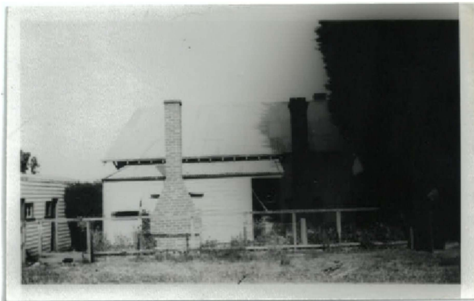
Figure 16 'Victory' House after the alteration of the roofline and addition of skillion kitchen and new external chimney (post c1933). Note skillion/flat roof and weatherboard cladding on adjacent north west outbuilding
