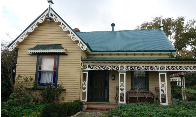
Figure 14. Original front (east) façade of Mossmont. (Landmark Heritage, 2022)
