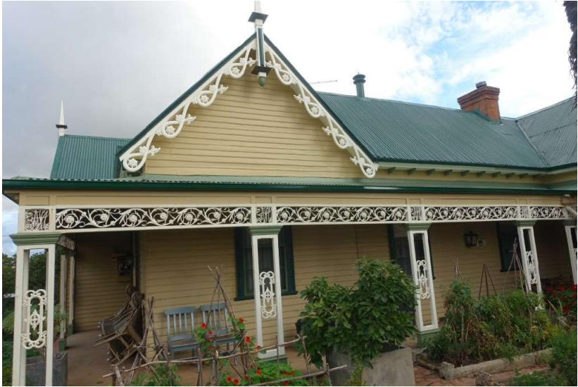
Figure 15. Early (east) end of the north elevation. The division between the first and second stages of the house is just left of the gable. (Landmark Heritage, 2022)
