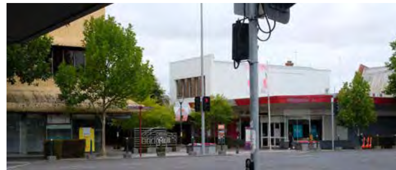
Sub-Area 1: Bridge Mall Gateway entrance view from Sturt Street
