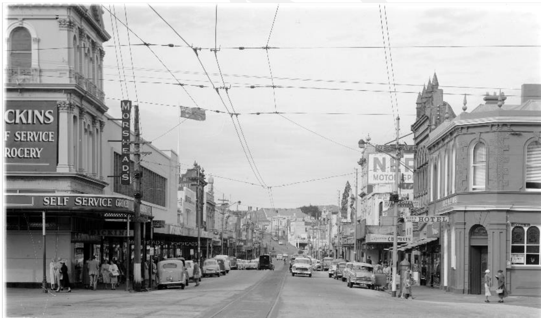
Figure 9. Looking east up Bridge Street from Sturt Street, c1950s (SLV, Rose Series P10709, Image H32492/7418).
