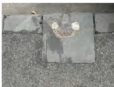
Figure 23. (right) Large kerb block with remnant marks where a verandah post was fixed (City of Ballarat, January 2023).
