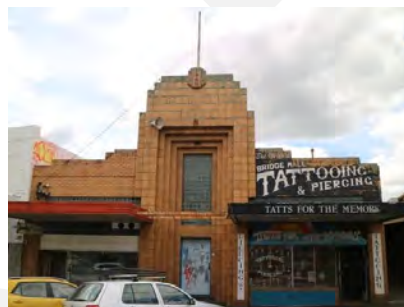
Figure 28. (left) Former North Grant Hotel, 3 Peel Street (GJM Heritage, November 2021).
