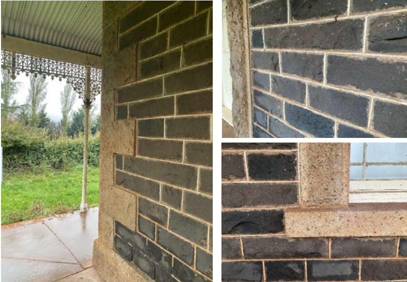
Tuckpointed bluestone, granite quoins and window surrounds
