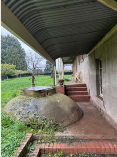
The brick cistern and water pump
