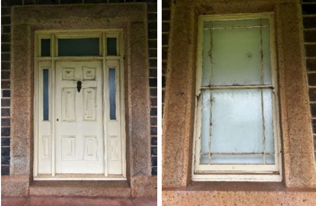
The timber door and window on the Western façade and granite surrounds
