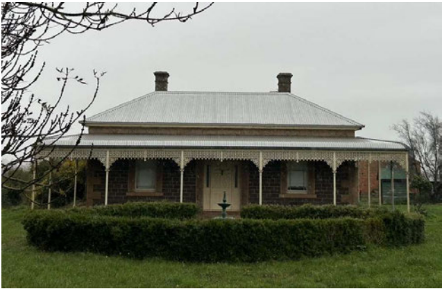
Lintel Grange, the front facade on a site visit on 24/05/2023 observed as pictured.
