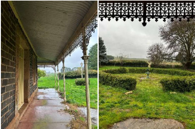
Cast iron posts on the Western facade
