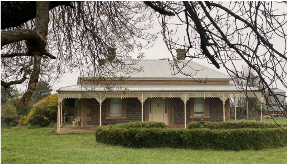
The front façade
