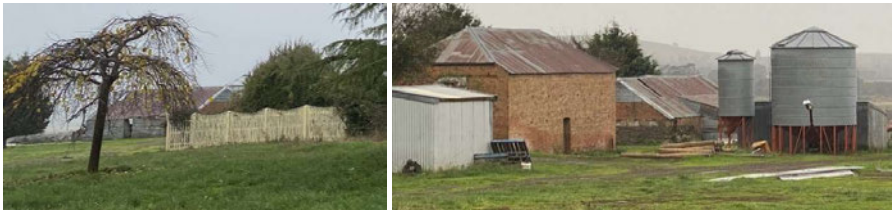
Left: Rear of dairy/ cow shed; Right: Dutch gable brick building and iron roofed stone and brick dairy in the back
