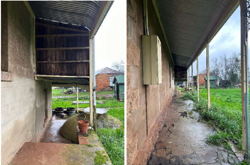
The Southern elevation looking towards East.
