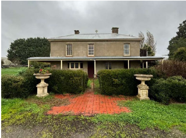
Lintel Grange, the rear elevation on a site visit on 07/06/2023 observed as pictured.
