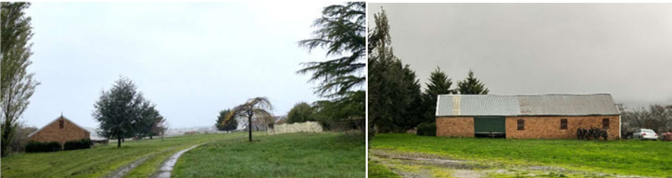
The brick barn
