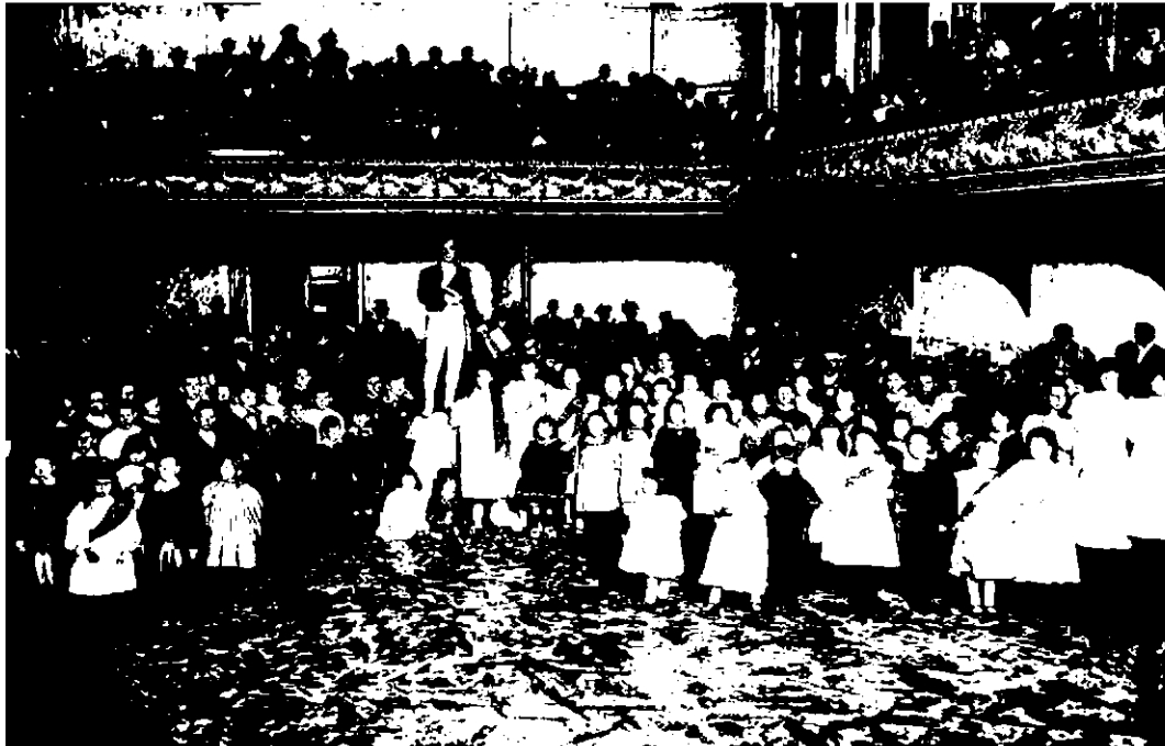
View of theatre interior with flat floor and single balcony level c1896
