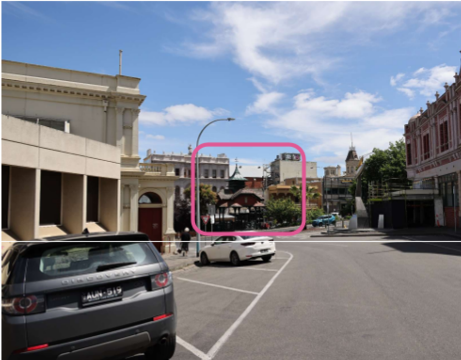
Figure 7 Photograph from Camp Street. The top of the north stair is visible including the eastern elevation with some limitation due to the angle.
