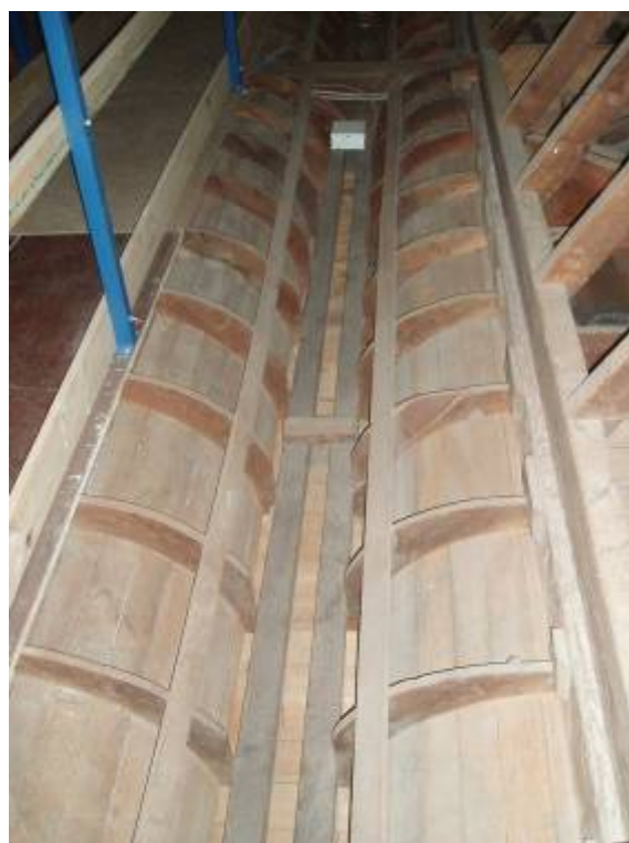
General views of the Roof Space
