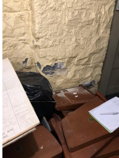
Photo 14 – Offices foyer wall does NOT have lead containing paint
