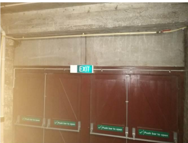
Photo 5 – Basement Auditorium fire escape fibro cement infill panels above exit doors
