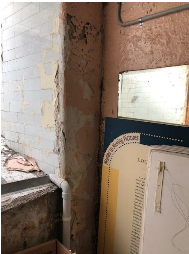
Photo 15 – Candy bar store wall has lead containing paint
