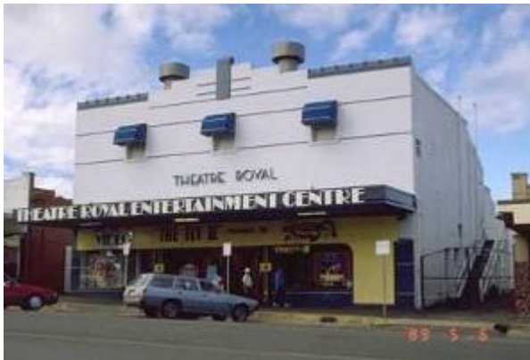
View of Theatre Royal, Castlemaine, 1989 (Source: Dep. for Env. and Heritage rt47182)
