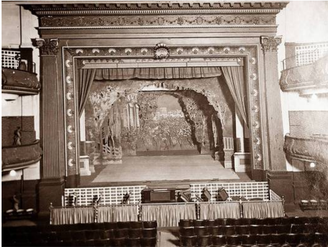
View of theatre interior in 1930
