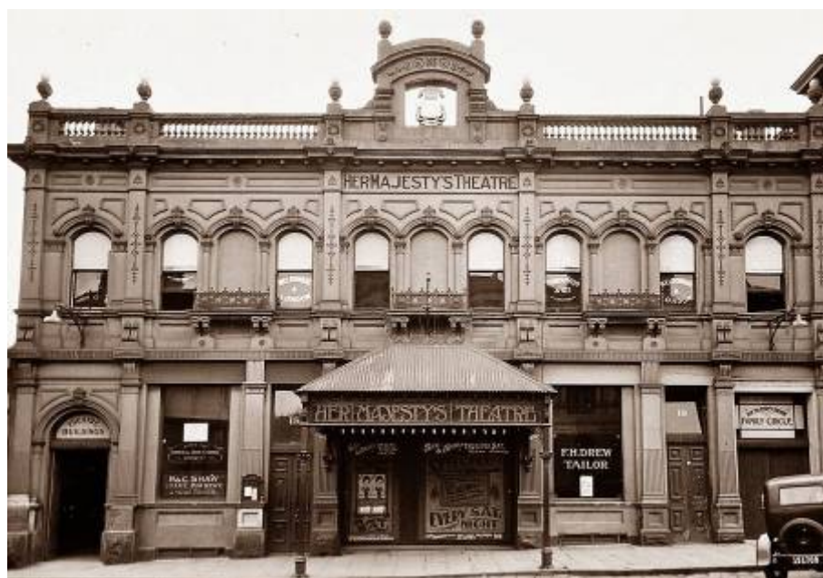
View of theatre in 1930 showing changes to central entrance including the 1912 portico (Source: Her Majesty's Archives, photo by Alec Hannah)
