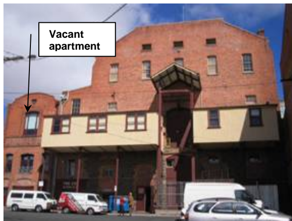
View of adjacent apartment
