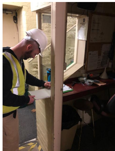
Photo 12 – Sub basement ticket booth door frame does NOT have lead coated paint
