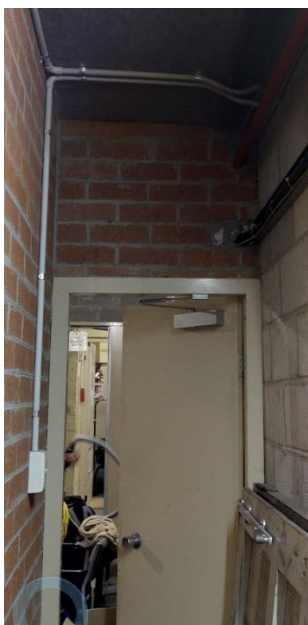
Switchroom Egress Door – Basement Level 1
