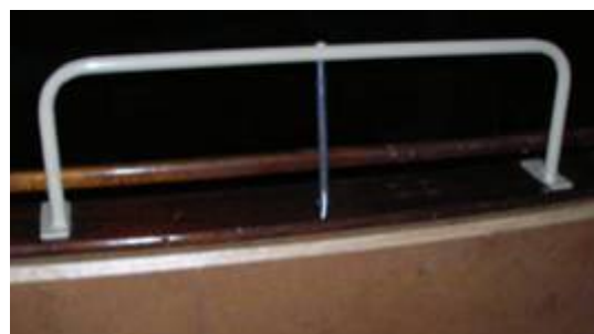
View of existing hand rail
