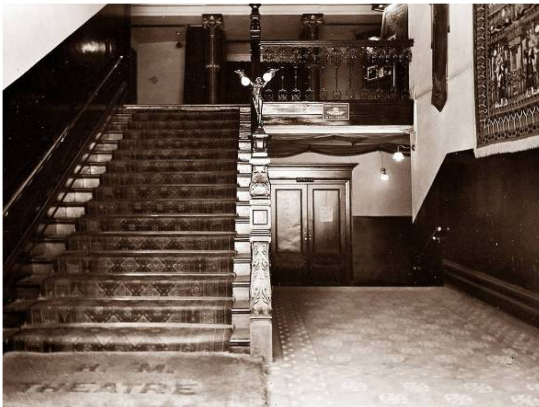
View of central entrance foyer in 1930
