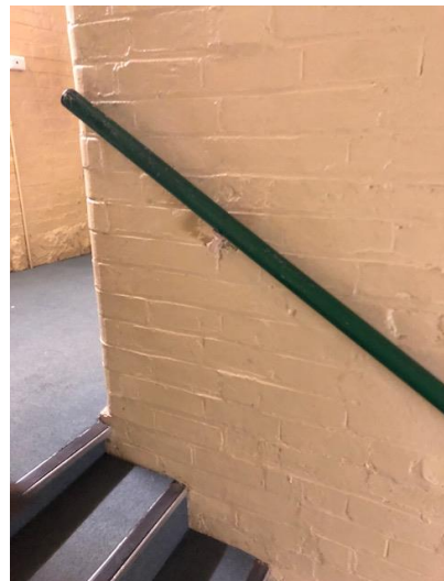
Photo 10 – Stage stairs do NOT have lead paint
