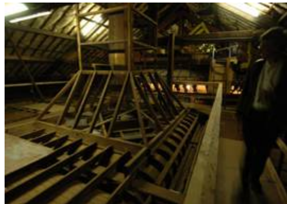
View of ventilation shaft (Source of photo: Jeremy Bannister)
