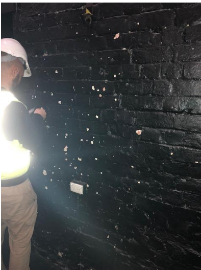
Photo 9 – Stage wall does NOT have lead paint
