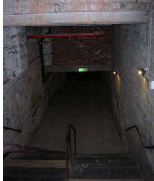
View of fire escape (121)
