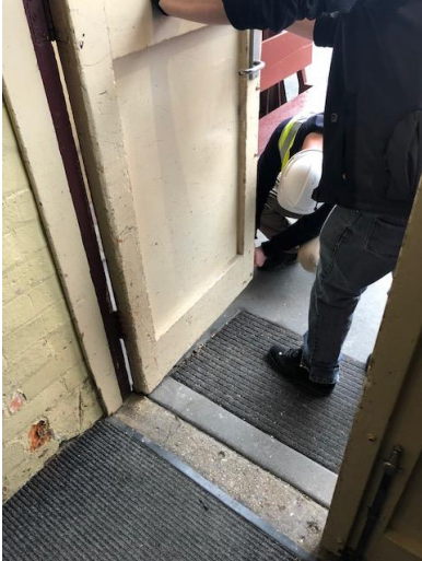
Photo 13 – Sub basement stage door does NOT have lead containing paint
