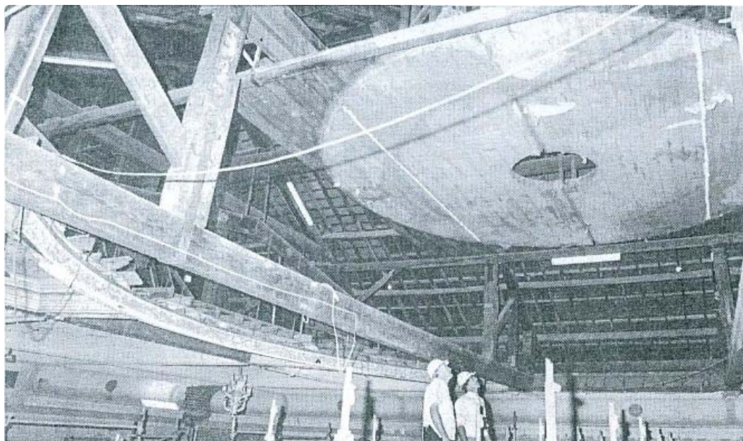
View of roof during reconstruction of dome in 1989
