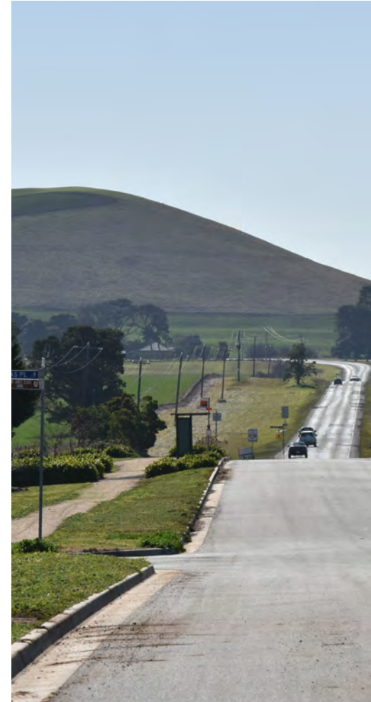
Creswick Street, Miners Rest: view of Mt Blowhard to the north
