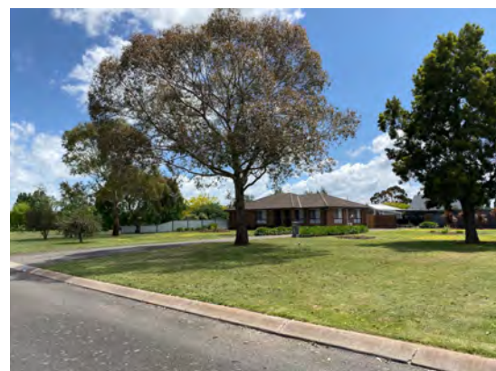
Dwelling in Burr Street, Sample Area 2
