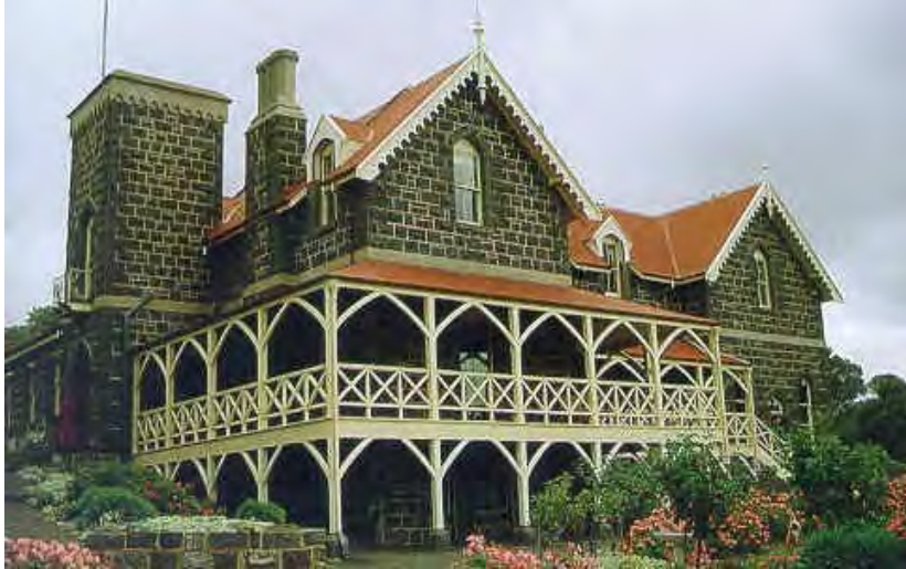
Figure 27. Elcho Homestead. Lovely Banks. Note the cusped gable bargeboard.
