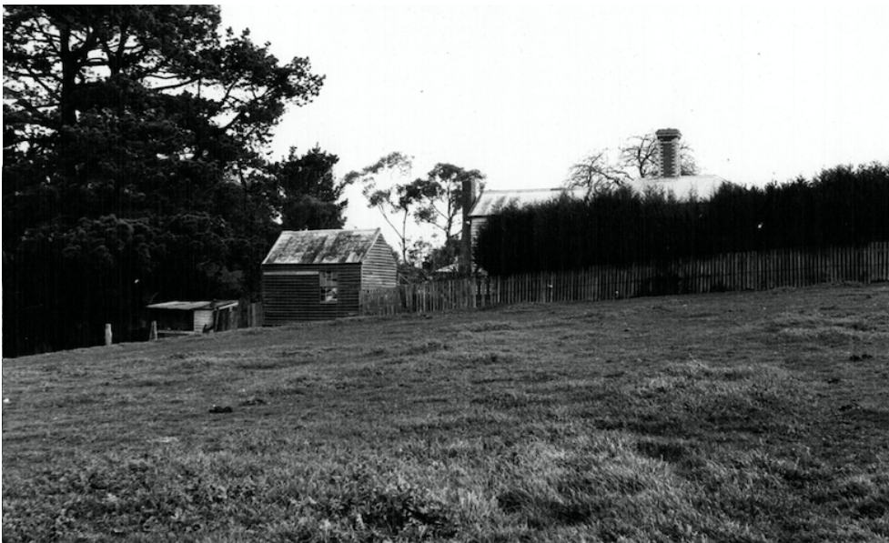
Figure 6. Views of the north-east side subject property in 1972-73 before renovation. Note the picket fence and hedging to the right, and gabled outbuilding to the left (since demolished). (Photos by Peter Cuffley 1972-73)
