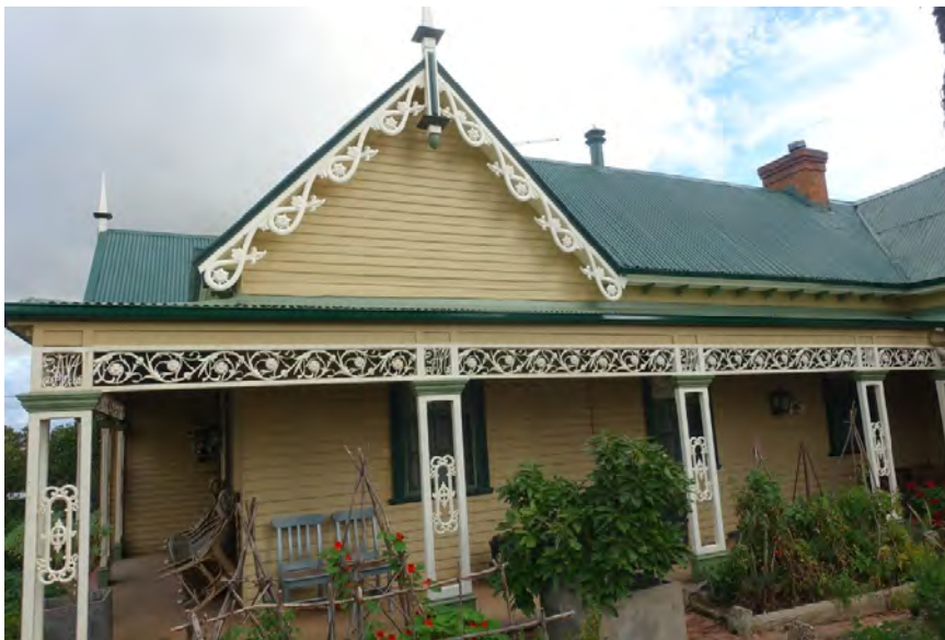
Figure 15. Early (east) end of the north elevation. The division between the first and second stages of the house is just left of the gable. (Landmark Heritage, 2022)
