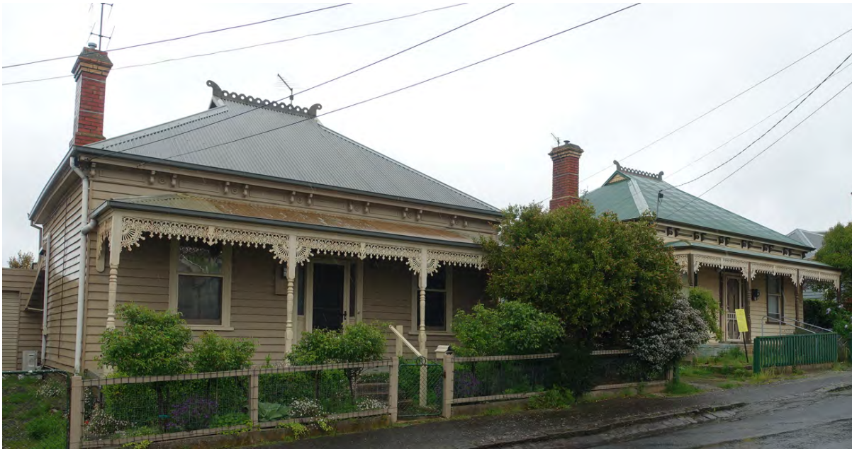
Image 2 - The identical houses at 15 & 17 Holmes Street, Source: Landmark Heritage 2022
