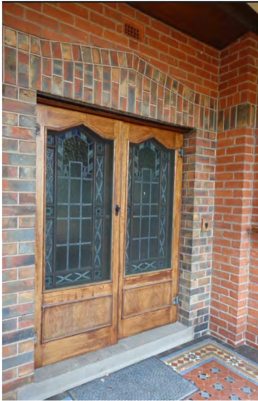
Figure 6. Glazed front doors, behind matching screen doors. (Landmark Heritage, 2022)
