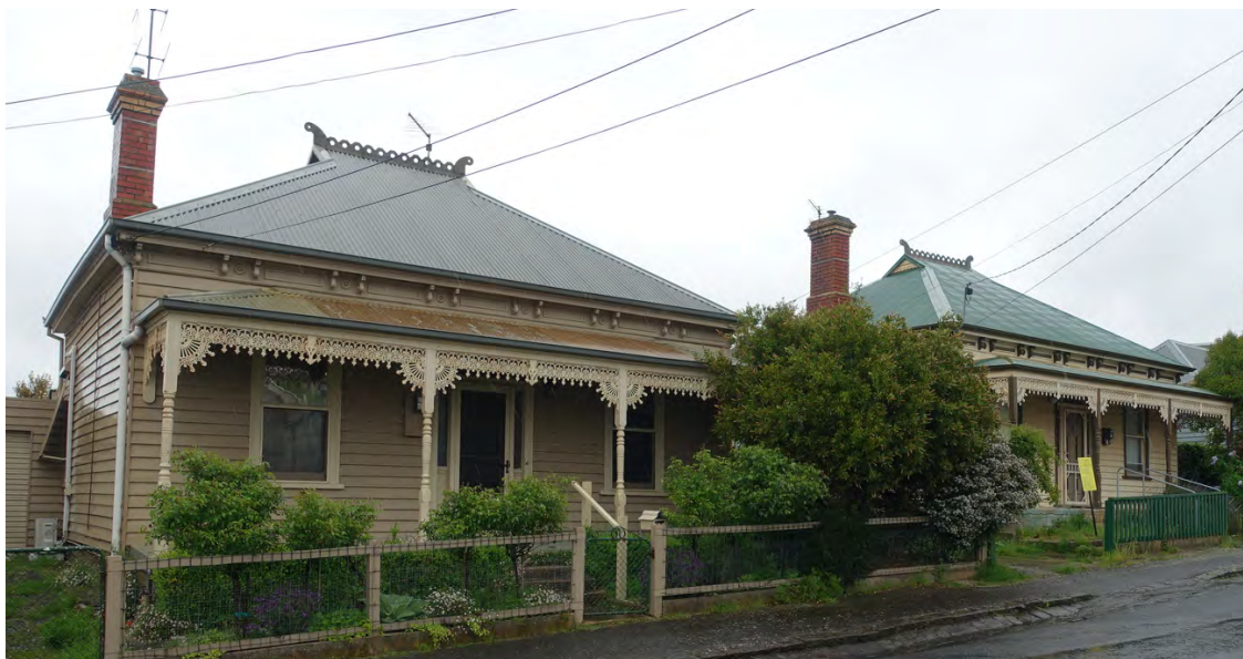
Figure 12. The identical houses at 15 & 17 Holmes Street, No. 17 (and likely 15) built by Coltman in 1903-05. (Landmark Heritage 2022)
