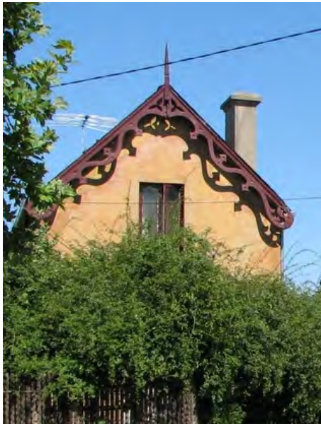
Figure 28. Bargeboard of 39 Nicholson Street, Abbotsford. (Heritage Victoria, 2008)
