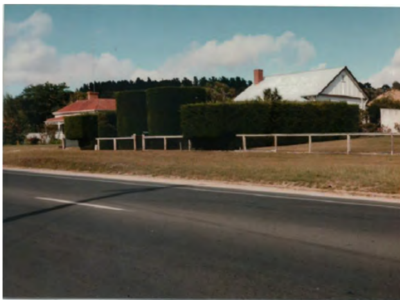
Figure 8. A view of the Chung house in 1986. (Source: Bindy Trembath 2022)
