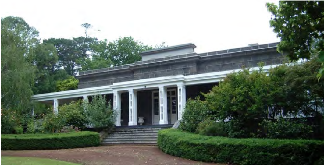
Figure 17. Maretimo, Portland North, built c1854. (Heritage Victoria, 2008)
