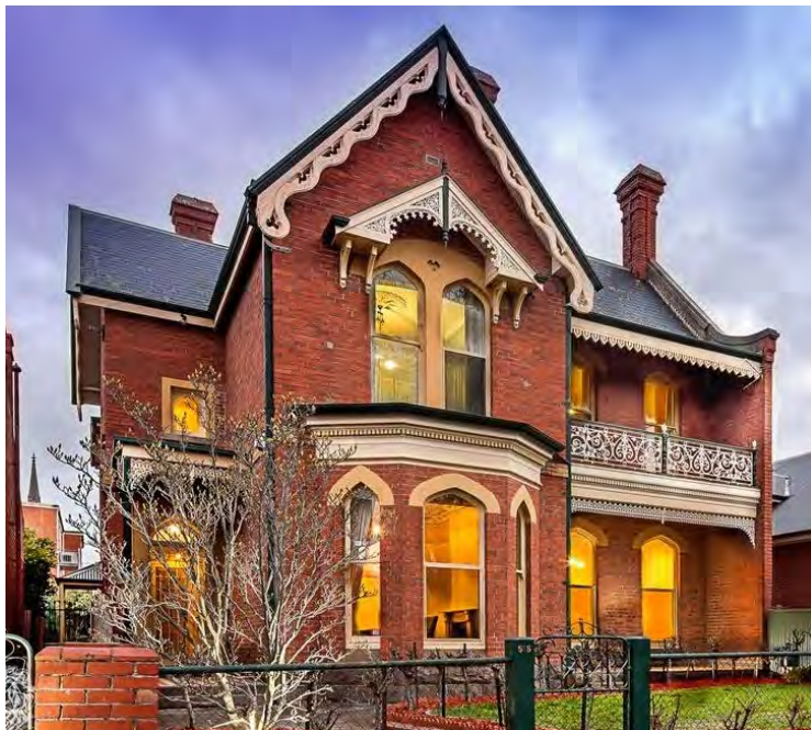
Figure 16. Former Congregational Church Manse, Ballarat Central. (realestate.com.au, 2020)
