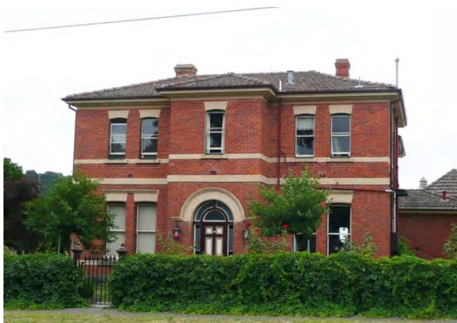
Figure 17. Former Female Refuge. (Heritage Victoria, 2008)
