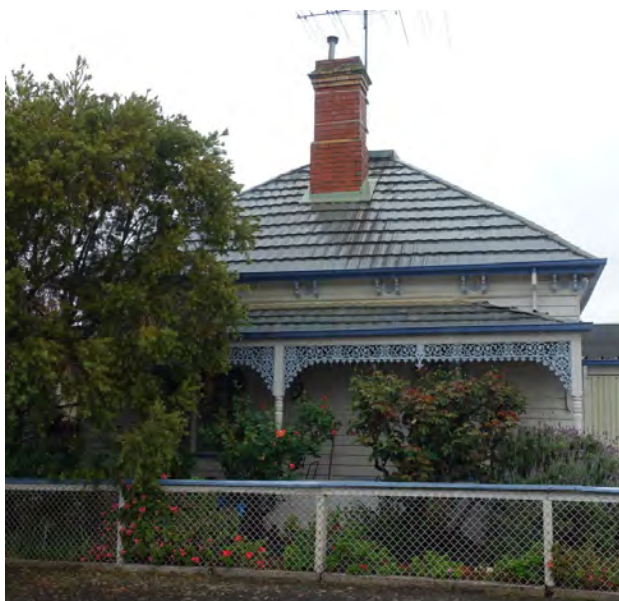
Figure 13. The 1904-05 house at 7 Holmes Street, built by Coltman. (Landmark Heritage 2022)
