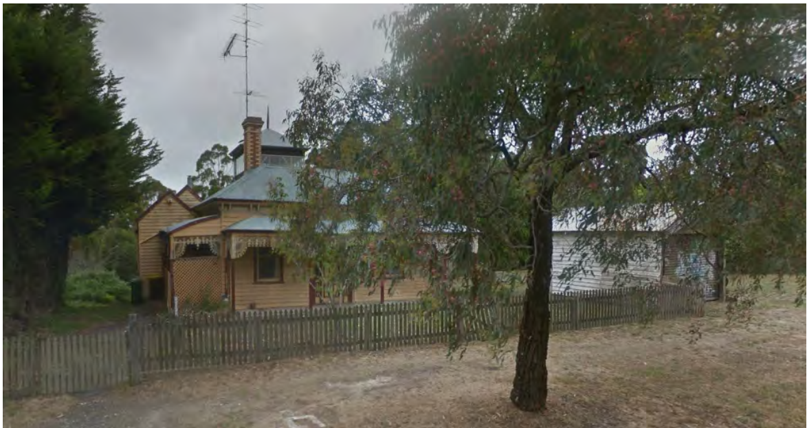
Figure 1 – Frontage of 89 Magpie Street, Golden Point, Source: Google Maps (Dec 2014)
