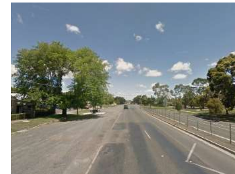
Top: Water Street Ballarat , shows the impact of powerlines on tree growth.
