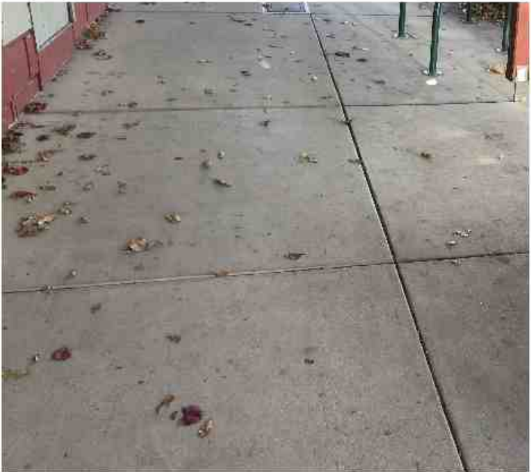
Grey concrete with tool joint - Ensure grey concrete matches this Warrenheip Street example.
