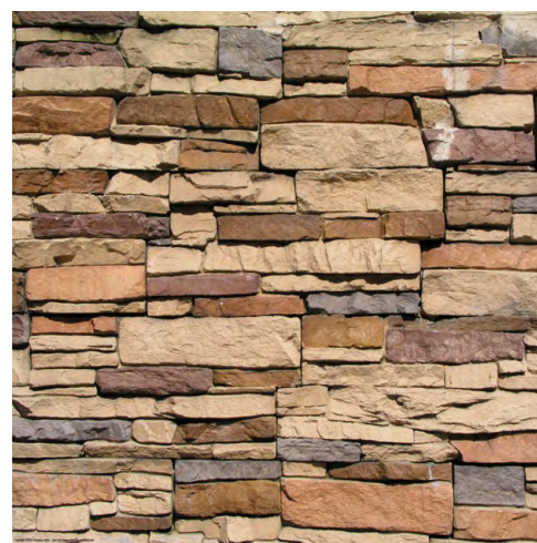
MAS-02 DRY STONE WALL - STRATA PATTERN CASTLEMAINE - LOCAL YAPEEN STONE
