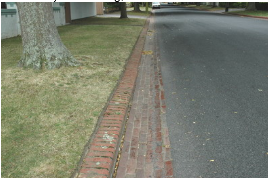
Photo 3.13: Detail of original brick kerb and channel, Colpin Avenue.
