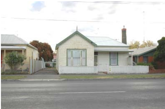
Photo 3.23: Edwardian styled dwelling, 104 Barkly Street, with capped timber picket front fence.
