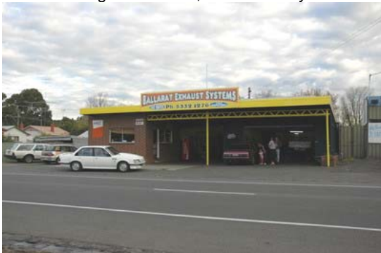
Photo 3.15: Ballarat Exhaust Building, 44 Eastwood Street.
