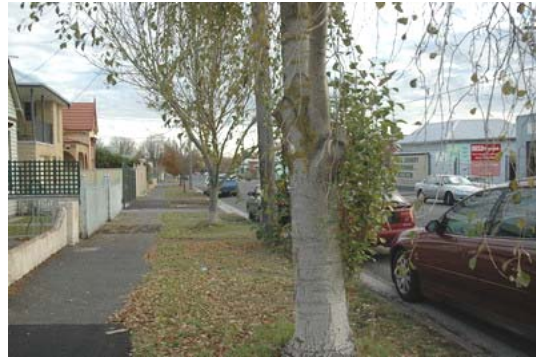
Photo 3.18: Asphalt footpath, grassed nature strips and concrete kerb and channel, Humffray Street.
