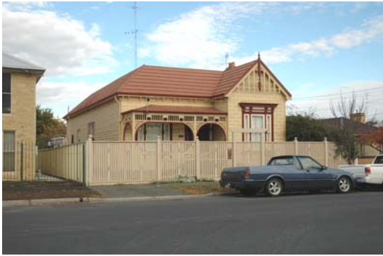
Photo 3.09: Edwardian styled dwelling (with introduced tiled roof), 109 Humffray Street.
