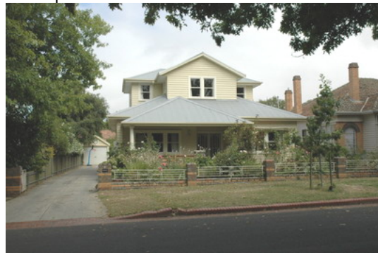
Photo 3.06: Interwar Bungalow styled dwelling with hipped roof front verandah (the two storey component represents later additions), 3 Colpin Avenue.
