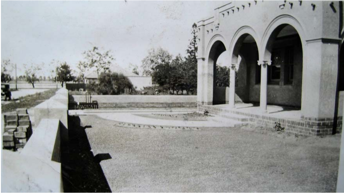
Figure 2.28: Front garden recently laid out at the “All Electric House”, 1933. Source: Bruce and Mary Green collection provided by Jennifer Burrell, Colpin Avenue, June 2005.
