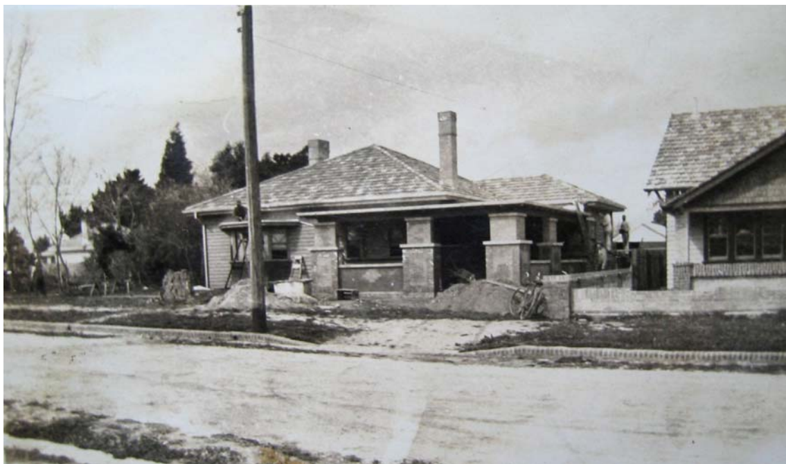
Figure 2.36: “Gas Feature” Home under construction, 1933. Also note the recently-constructed brick kerb and channel. Source: Bruce and Mary Green collection provided by Jennifer Burrell, Colpin Avenue, June 2005.
