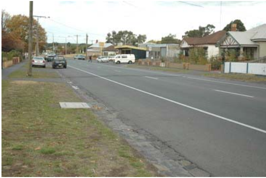
Photo 3.17: Eastwood Street, showing recently constructed bluestone spoon drains.
