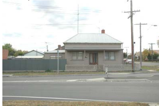
Photo 3.04: Rudimentary Late Victorian styled dwelling with introduced front flat roofed verandah, 202 Barkly Street.
