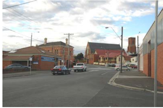
Photo 3.28: View north from Humffray Street to St. Paul's Anglican Church and Post Office, Bakery Hill.
