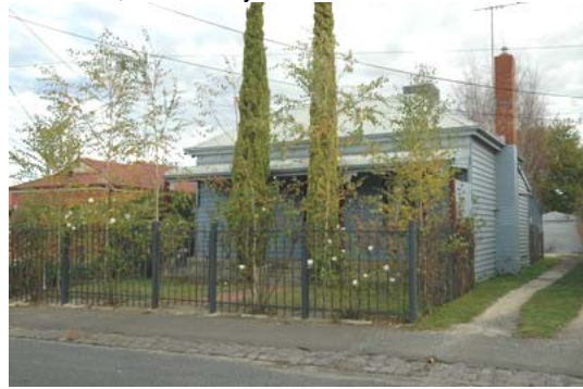
Photo 3.06: Late Victorian style dwelling at 13 Porter Street with face red brick interwar chimney (soldier course top), suggesting that it may have been relocated to this site.
