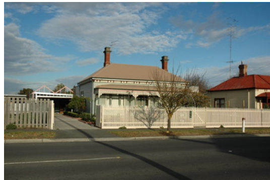
Photo 3.22: Late Victorian styled dwelling, 203 Humffray Street, with pointed timber picket front fence.
