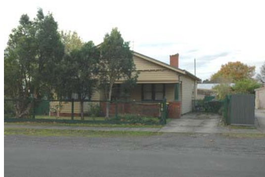
Photo 3.24: Interwar Californian Bungalow styled dwelling, 25 Steinfeld Street, with timber post and woven wire fence.
