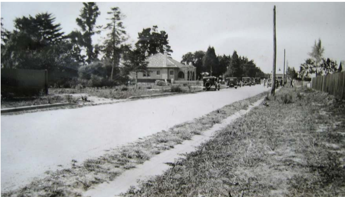
Figure 2.39: Streetscape view of Colpin Avenue looking north with the “All Electric House” in the background, 1933. Note the brick kerb and channel that had been constructed by this time and the laid out nature strips with graveled pedestrian tracks (the grass had not been planted by this time). Source: Bruce and Mary Green collection provided by Jennifer Burrell, Colpin Avenue, June 2005.
