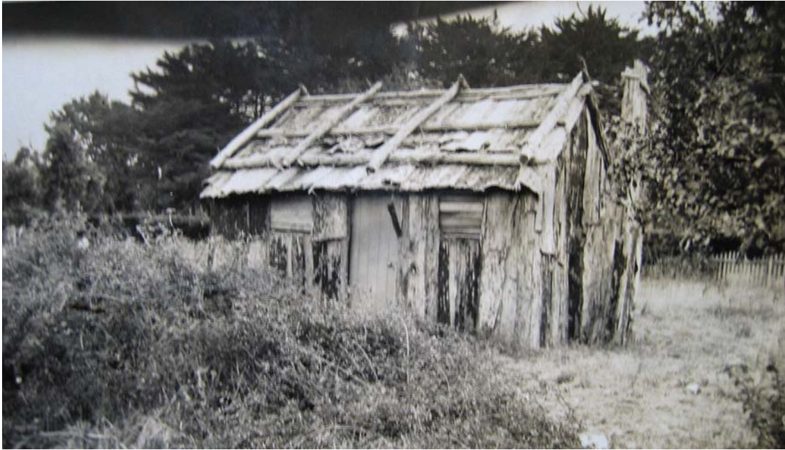
Figure 2.18: Replica of slab and bark pioneer's cottage used as the Ideal Homes Exhibition Office, dated either before or after the exhibition in 1933. Source: Bruce and Mary Green collection provided by Jennifer Burrell, Colpin Avenue, June 2005.
