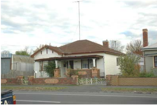
Photo 3.25: Interwar Bungalow styled dwelling, 40 Eastwood Street, showing early low solid brick front fence.
