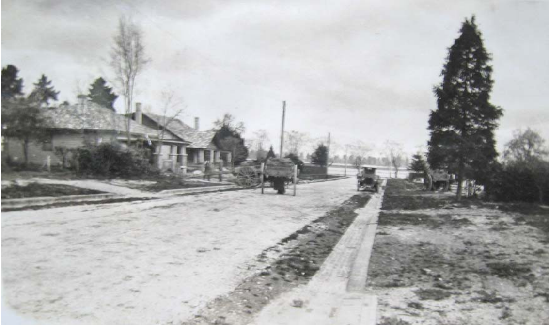
Figure 2.40: Streetscape view of Colpin Avenue looking south towards Lake Wendouree, 1933. The “Gas Feature Home” and other house built by David Quayle at 6 Colpin Avenue are shown in the background. Note the newly constructed brick kerb and channel, laid nature strips (with the grass yet to be planted) and the surviving Italian Cypress tree that appears to have been temporarily retained. This tree may have formed part of Smith’s Nursery that had previously taken up the Colpin Avenue area. Source: Bruce and Mary Green collection provided by Jennifer Burrell, Colpin Avenue, June 2005.
