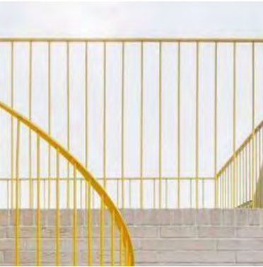
BA3 - Coloured metal rod balustrade
