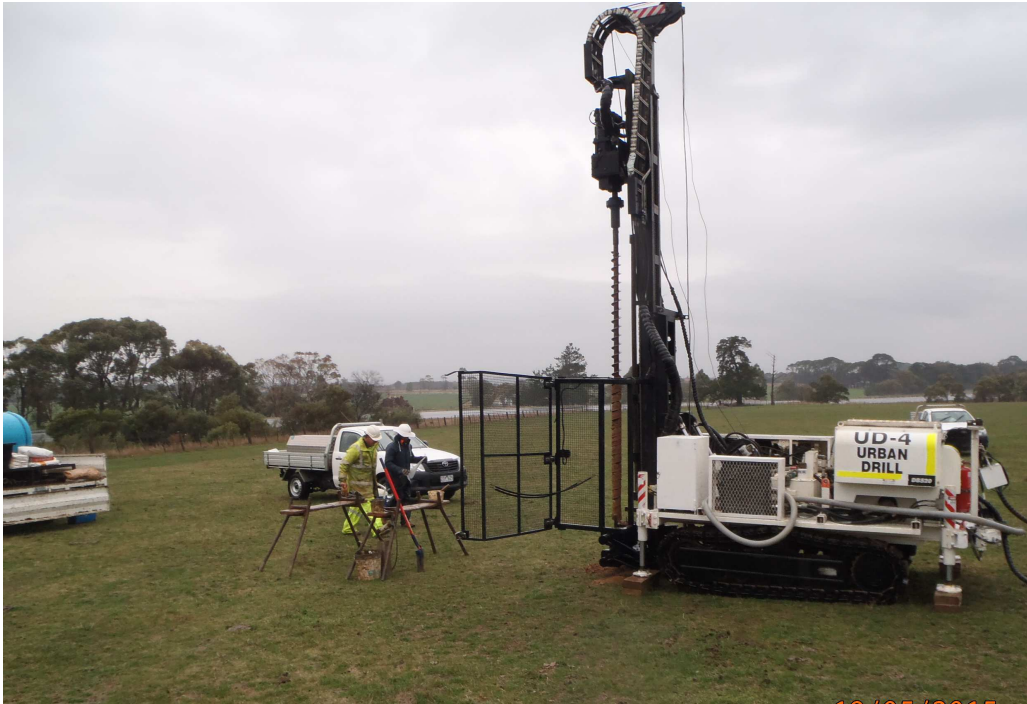
Photo 1 – Drilling borehole MW103.
