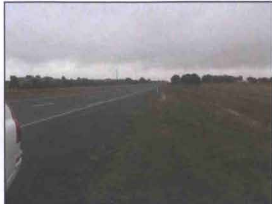
Figure 8: Western Highway - view west
