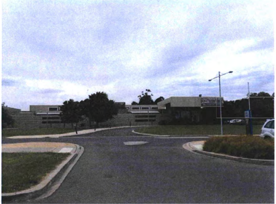
Photo 4: Exterior of Clubhouse from car park
