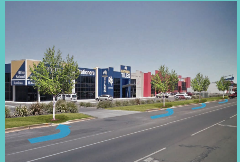
Stormwater drainage to water street trees in new developments
