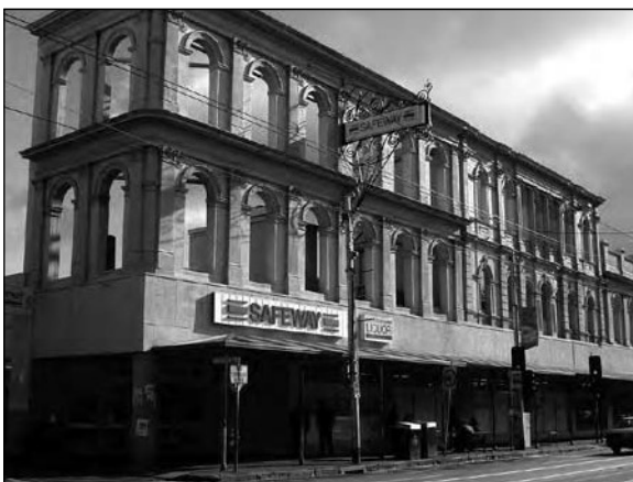
Facadism resulting from inadequate fabric retention
