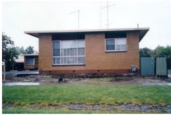
Figure 72. Poor maintenance / lack of front gardens.
