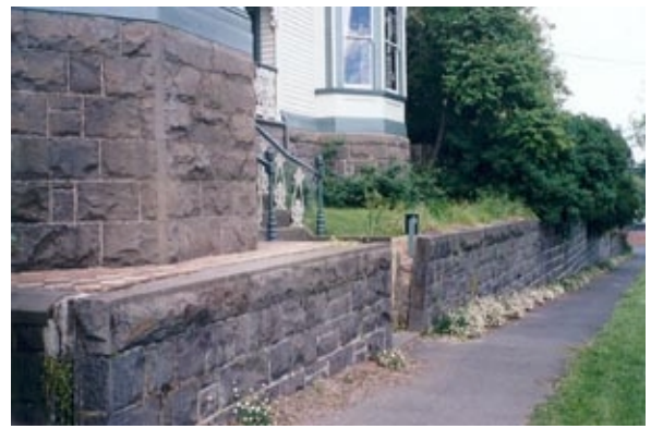
Figure 54. Historic bluestone retaining wall / fence.
