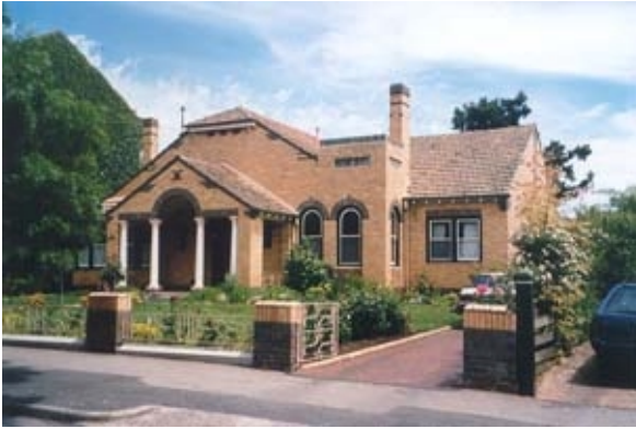
Figure 30. Typical Inter-war (1915-1945) brick building in Lyons Street North.
