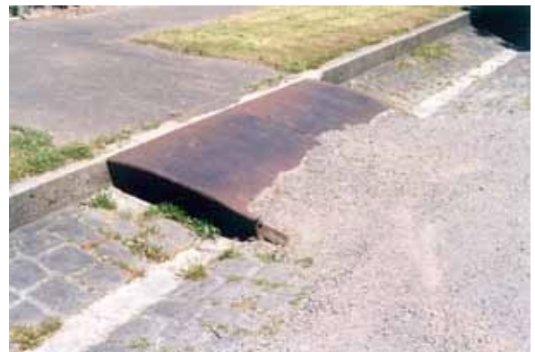
Figure 19. Metal bridge (arched) in Kent Street.
