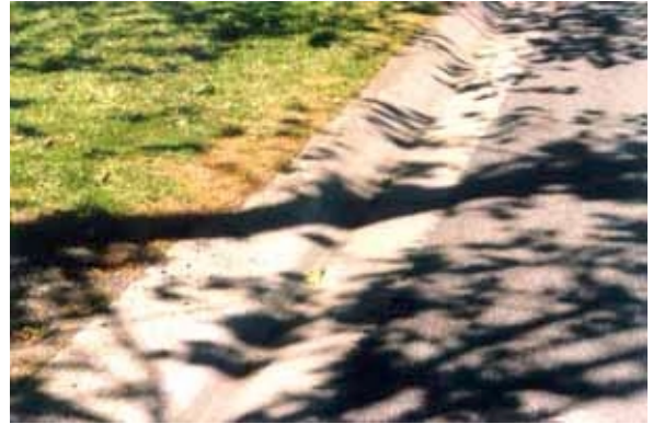
Figure 3. Integrated concrete kerb and gutter (roll over type) in Forest Street.
