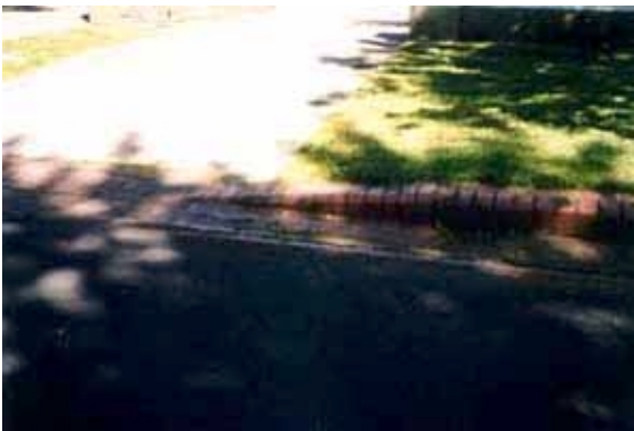
Figure 12. Bullnose brick kerb and brick spoon drain in Colpin Avenue.
