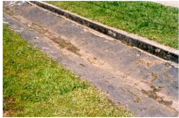
Figure 11. Bluestone pitcher spoon drain gutter with concrete upstand in Dowling Street.
