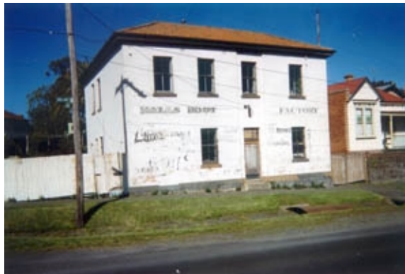
Figure 75. Halls boot factory building in Nolan Street.
