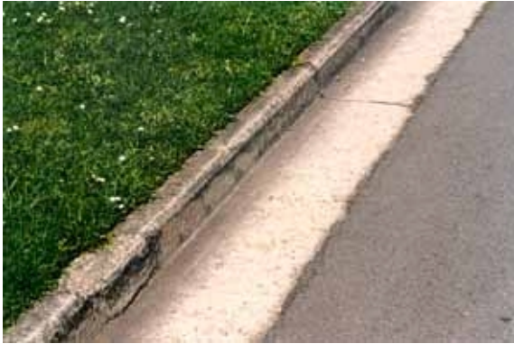
Figure 4. Integrated concrete kerb and gutter with wide invert in Haddon Street.
