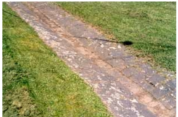
Figure 9. Bluestone pitcher spoon drain.
