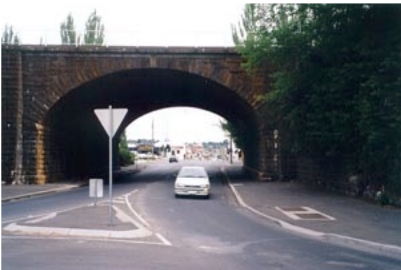
Figure 41. Landmark arched railway bridge in Peel Street.
