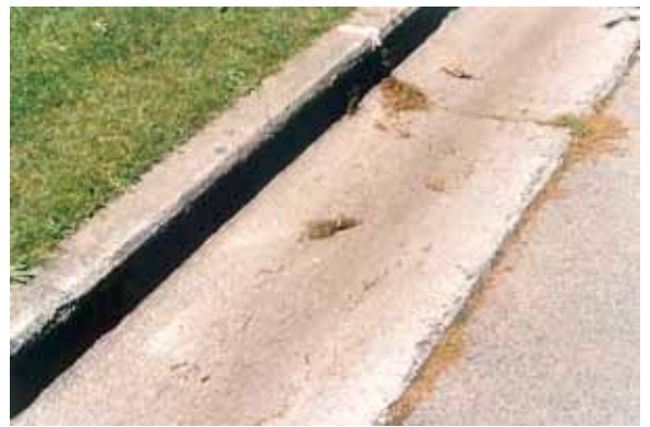
Figure 15. Integrated concrete kerb with concrete spoon drain gutter in Martin Avenue.
