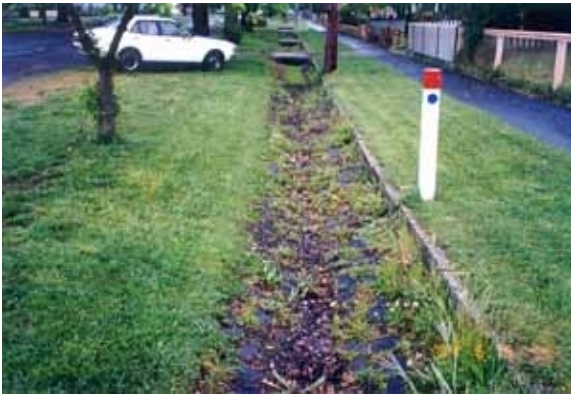
Figure 10. Bluestone pitcher channel drain in Clyde Street.
