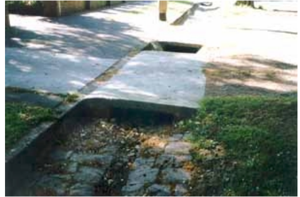
Figure 17. Concrete bridge (arched) in Russell Street.
