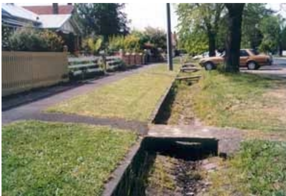
Figure 18. Concrete bridge (flat) in Talbot Street North.
