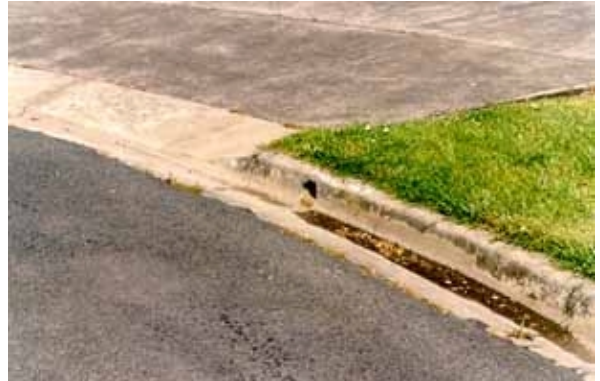
Figure 5. Integrated concrete kerb and gutter with narrow invert in Stafford Court.
