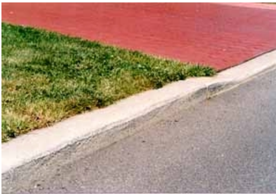
Figure 6. Concrete kerb only in Parade Court.
