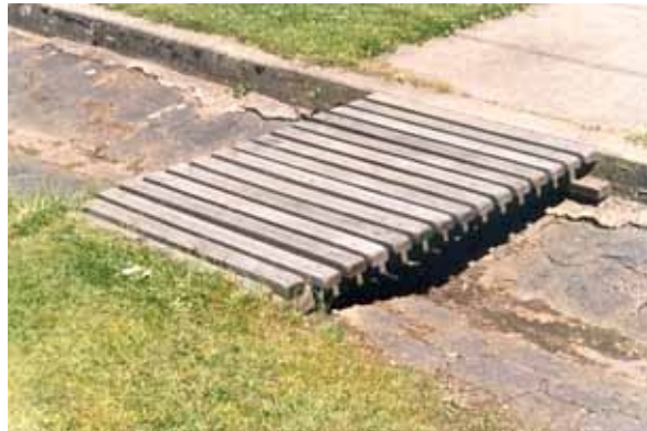
Figure 21. Timber pedestrian bridge in Dowling Street.
