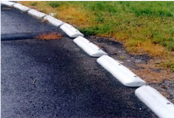
Figure 61. Inappropriate road edging.
