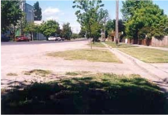
Figure 16. Bitumen or concrete at grade - example of concrete crossovers in Gregory Street.
