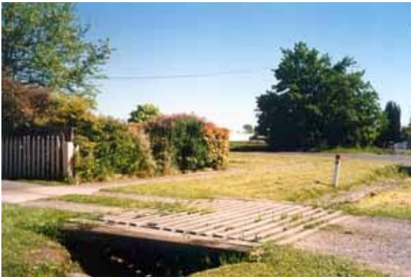
Figure 20. Timber bridge in Lexton Street.
