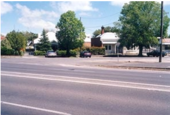
Figure 63. Poorly defined intersections are dangerous.
