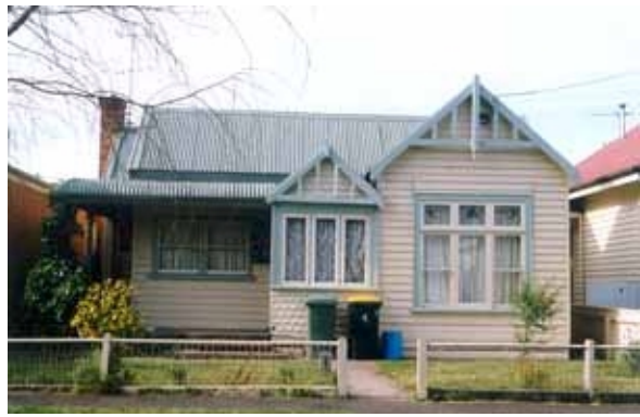
Figure 27. Typical Edwardian building (1900-1915) in Sussex Street.
