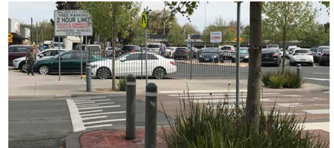
CROSSING ON LITTLE BRIDGE STREET BETWEEN BRIDGE MALL AND THE COUNCIL-OWNED CAR PARK
