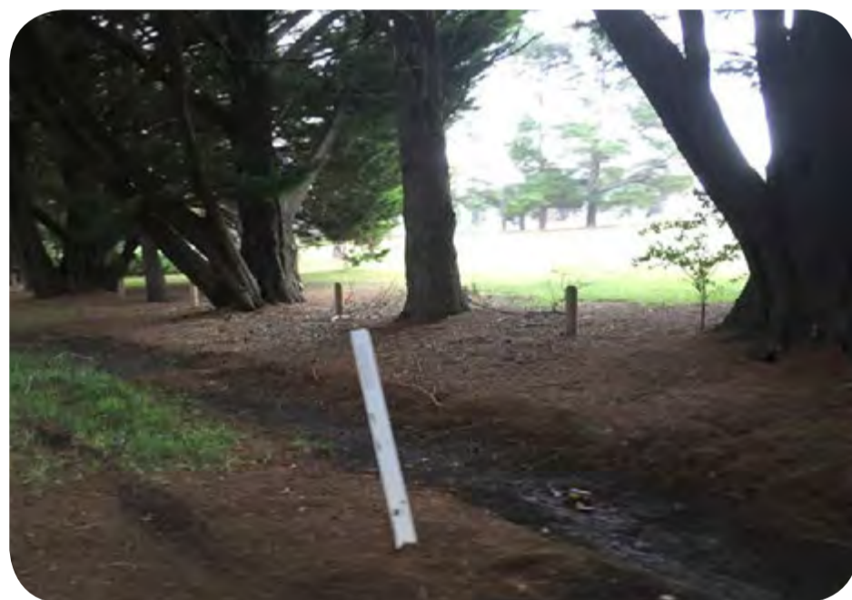
Roadside marker that has been hit by vehicle
