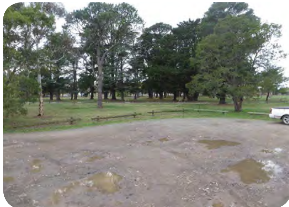
Unsealed car park
