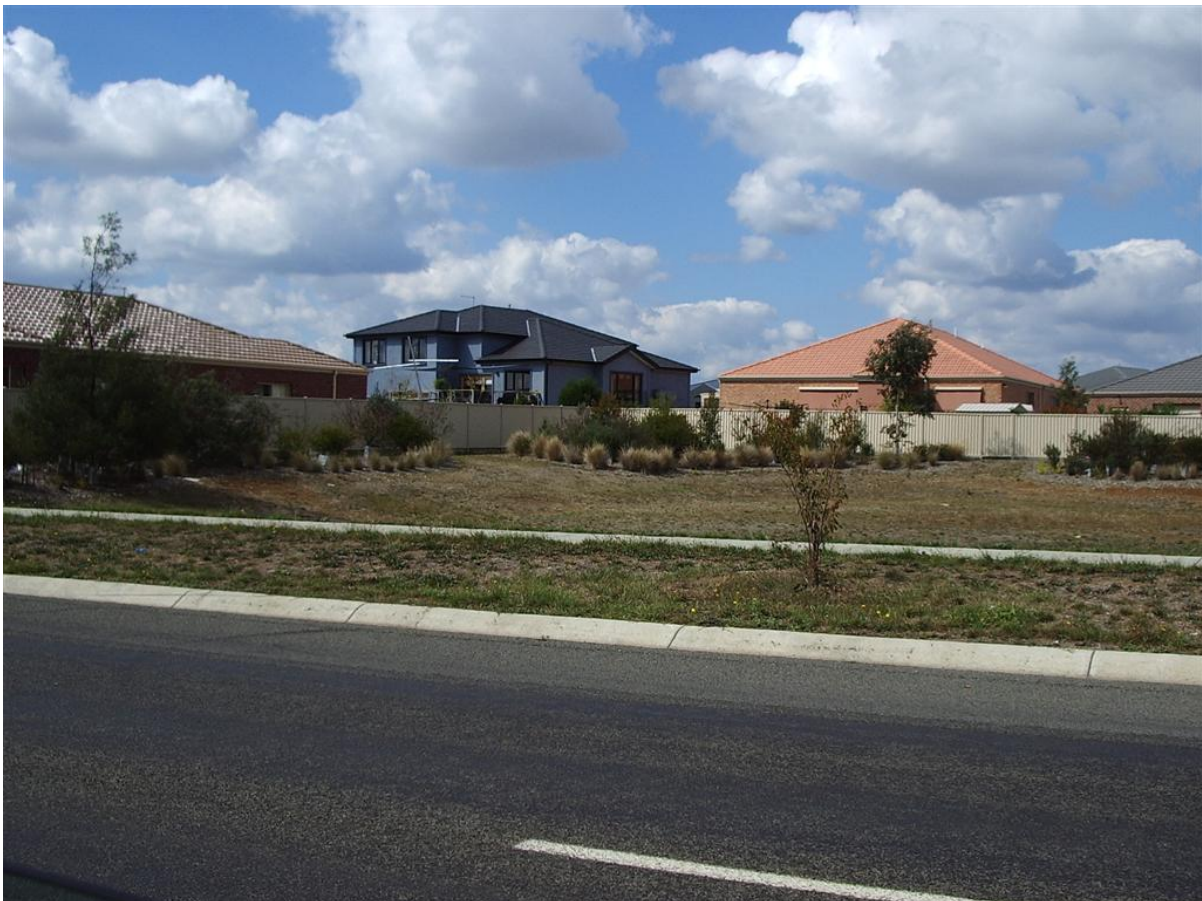
Dyson Drive Reserve in Alfredton – landscaped with local native vegetation with open spaces for passive play but primary function is a stormwater retention basin.
