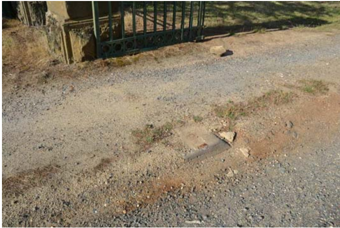
Photo 4 Detail of central stone slab for fastening gates
