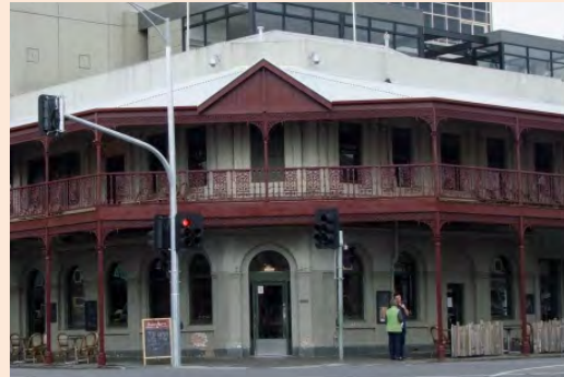
Above: The City of Ballarat's grant program has helped owners undertake large scale and small scale conservation works, including reinstatement of 'Jackson's' verandah in Lydiard Street.
