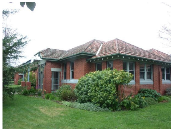
Building 1: Former Toddlers’ Block.
