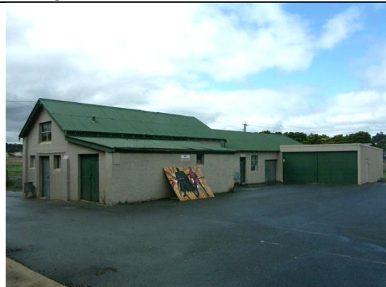
Building 3: Former Sloyd Room.
