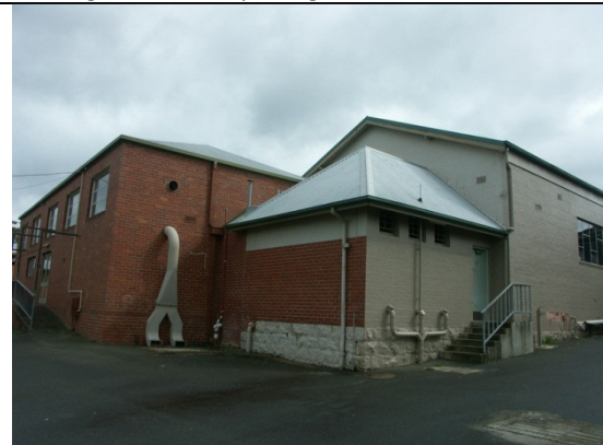
Building 8: Former Gymnasium addition (Service Block).
